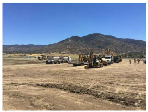
Figure 1 – Construction crews continued with soil import, grading, and compaction activities at the Banducci Substation, August 14, 2017.
