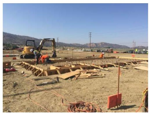
Figure 1 – Construction crews began foundation construction inside the Banducci Substation.
