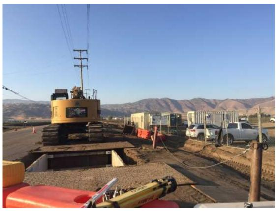
Figure 3 – Vault excavation for the underground subtransmission work along Pellisier Road.
