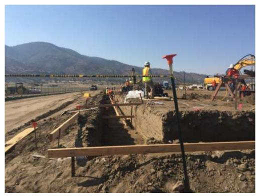
Figure 2 – Trenching for the perimeter wall foundation at the Banducci Substation.
