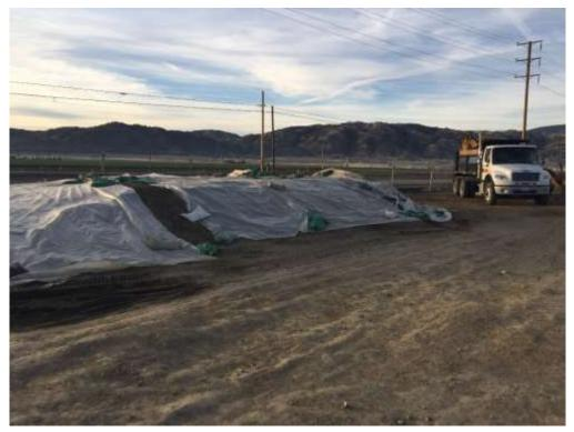
Figure 4 – Soil stockpile covered at the Banducci Substation to prevent erosion.
