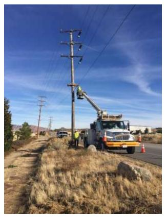
Figure 2 - Telecom crews installing fiber on existing poles along Highline Road, Route 1.
