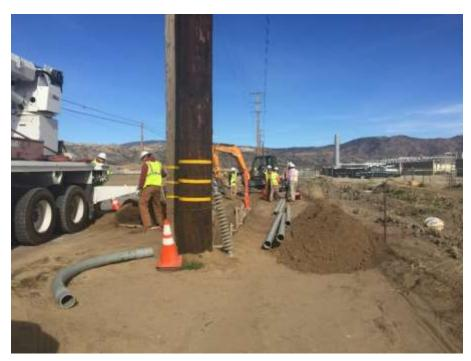
Figure 1 – Henkels and McCoy continue with trenching and conduit placement along Pellisier Road.
