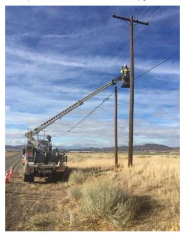
Figure 2 - Telecom crews installing fiber on existing poles near Highway 202.
