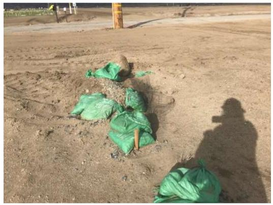
Figure 3 – Bird netting used to cover ends of conduit was left unsecured and became caught in perimeter sandbag berm causing a microtrash and wildlife entrapment concern documented by the CPUC EM on February 14.
