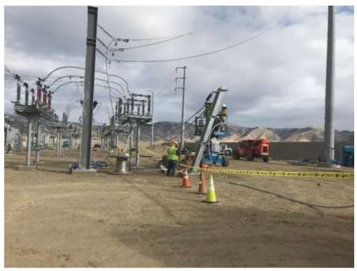
Figure 1 – Henkels and McCoy crew installing jumpers on the 66 kV rack.
