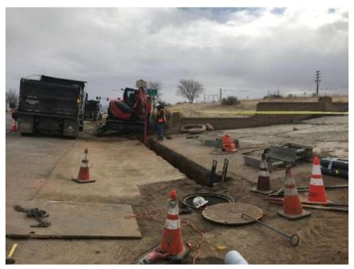
Figure 2 – Telecom underground crews trenching to tie in with overhead sections installed along Highway 202 and Woodford Tehachapi Road.
