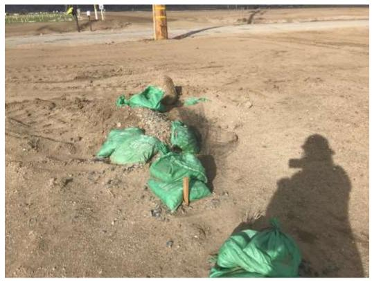
Figure 3 – Bird netting used to cover ends of conduit was left unsecured and became caught in perimeter sandbag berm causing a microtrash and wildlife entrapment concern, as documented by the CPUC EM on Feb 14.
