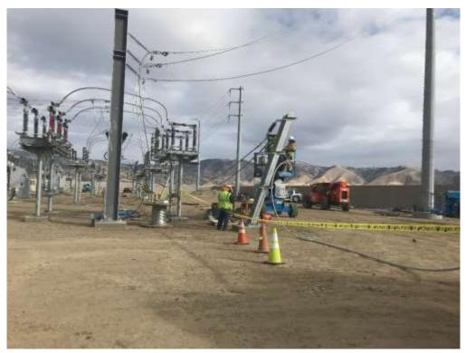
Figure 1 –H&M crew installing jumpers on the 66 kV rack.
