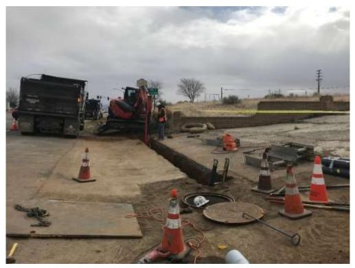
Figure 2 – Telecom underground crews trenching to tie in with overhead sections installed along Highway 202 and Woodford Tehachapi Road.
