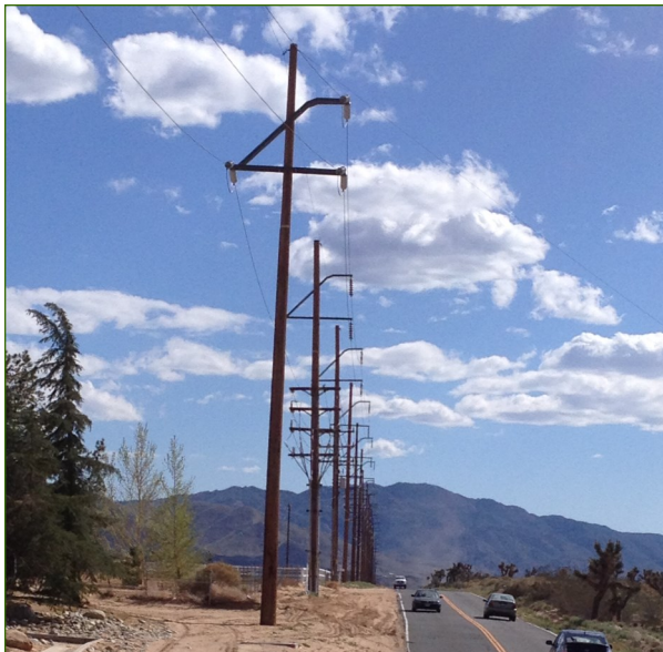
Subtransmission lines
