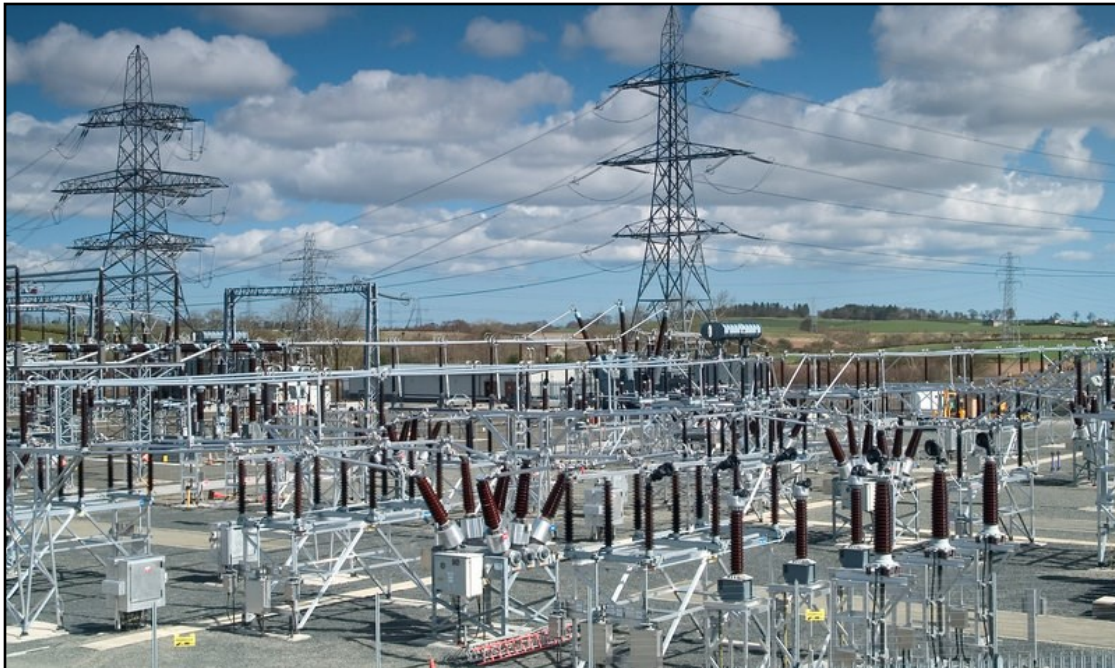
Electric substation, with transformers and associated equipment shown in the foreground, and transmission towers and lines present in the background. (photo credit: www.ethospower.in )
