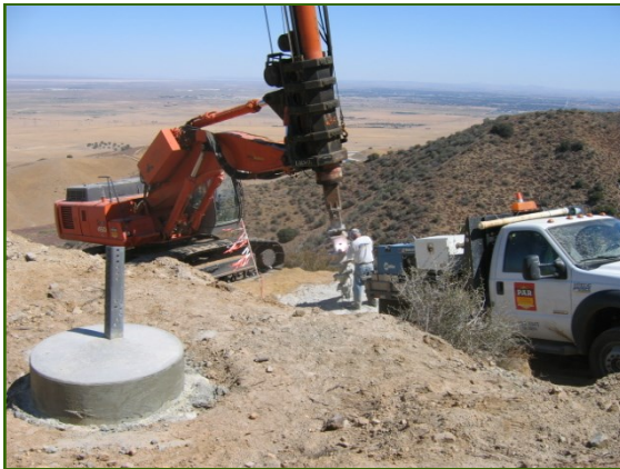
Foundation construction for an LST.
