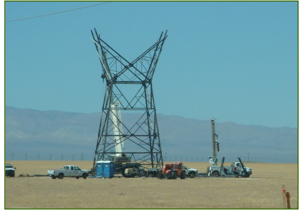
Transmission line tower construction site.
