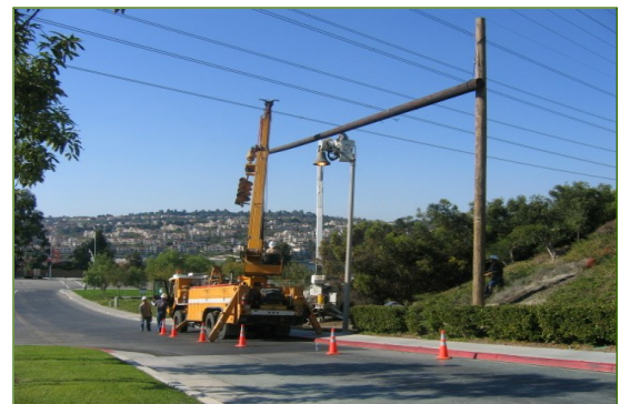
A guard structure being erected at a street crossing.
