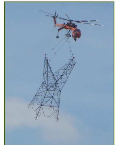
A sky crane helicopter carrying the top section of a LST.
