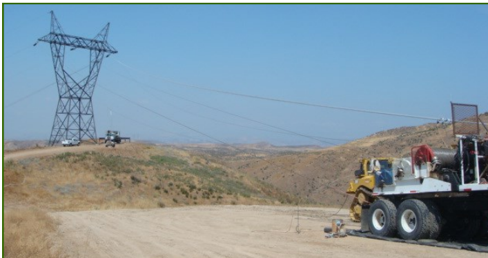
Pulling phase of a wire-stringing operation. Note the reel of conductor on the right side of the photo.
