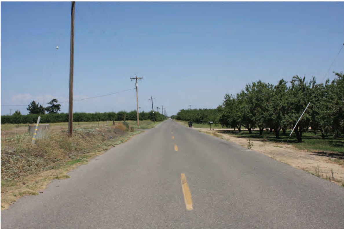
Photograph 6. View from Mercedes Avenue near Arena Way looking east.
