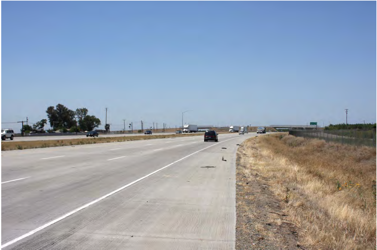
Photograph 9. View from Highway 99 near Liberty Avenue exit looking northwest.*
