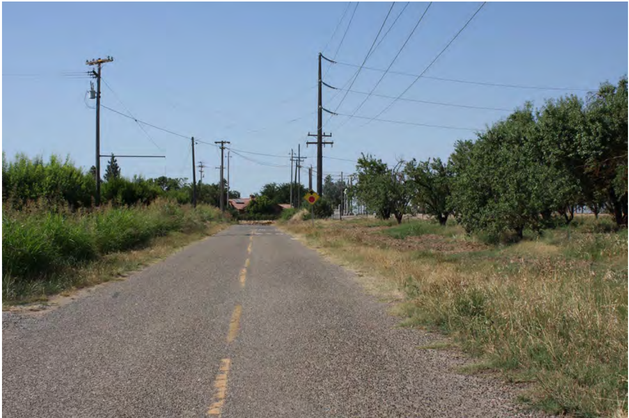
Photograph 3. View from West Lane looking north toward Cressey Substation.
