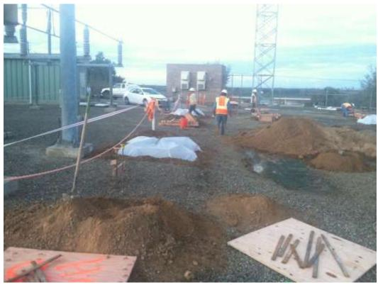
Figure 7 – Holes were securely covered at the end of each working day at the Cressey Substation. View north, December 4, 2014.
