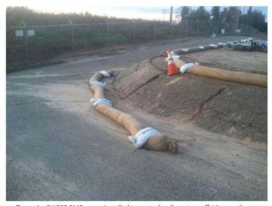
Figure 4 – SWPPP BMPs were installed to control sediment runoff. View northwest, December 4, 2014.
