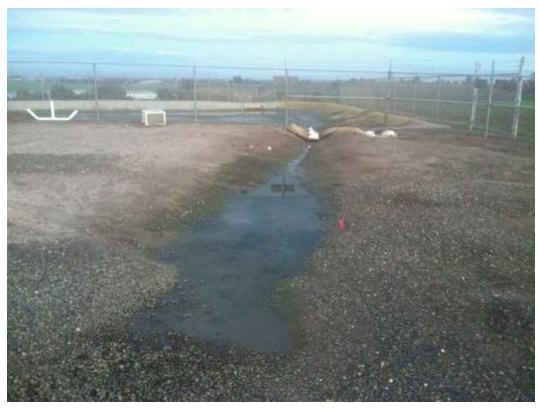
Figure 3 – SWPPP BMPs were installed to control sediment runoff. View east, December 4, 2014.
