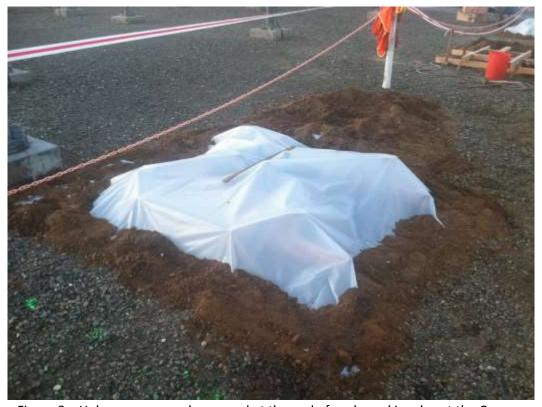
Figure 8 – Holes were securely covered at the end of each working day at the Cressey Substation. View northwest, December 4, 2014.
