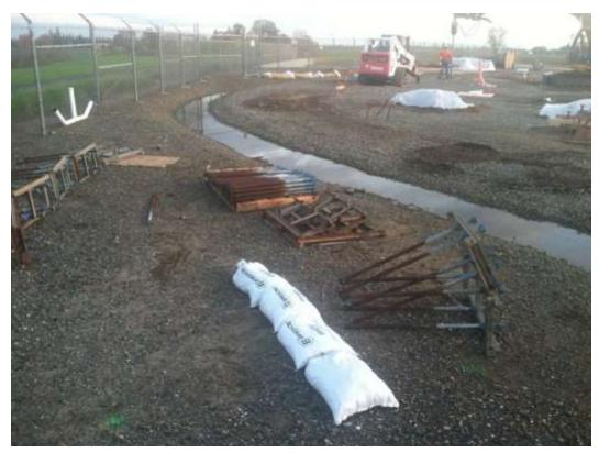
Figure 5 – SWPPP BMPs were installed to control sediment runoff. View southeast, December 4, 2014.
