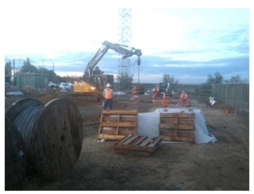
Figure 2 – Augering and trenching at the Cressey Substation occurred during the subject week. View north, December 4, 2014.
