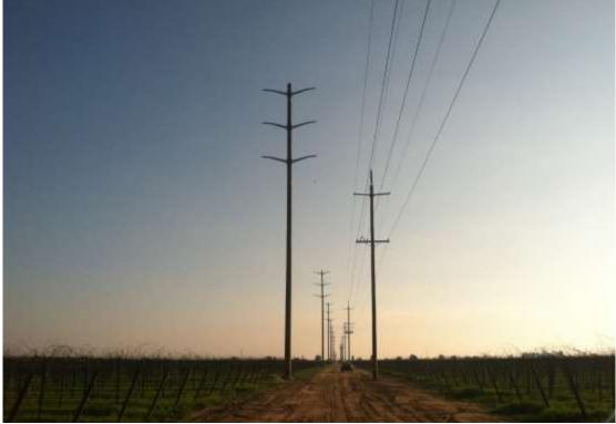
Figure 4 – Installation of new permanent poles (left) occurred adjacent to the temporary Shoo Fly poles (right). View south, 01/29/15.
