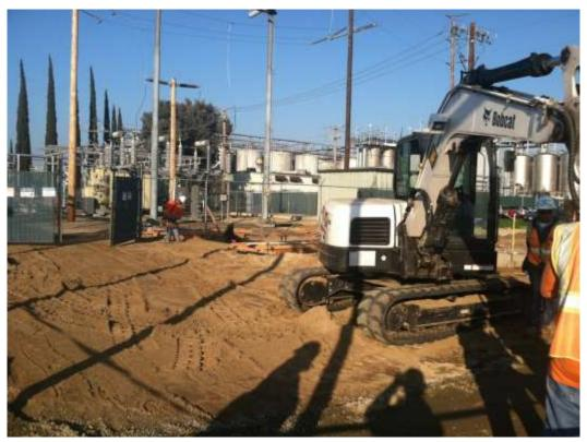
Figure 2 – Augering and foundation installation continued at the Gallo Substation during the subject period. View northeast, 01/29/15.
