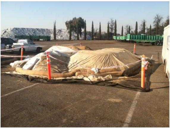
Figure 6 – Soil pile is properly contained at the Gallo work area. View northwest, 01/29/15.
