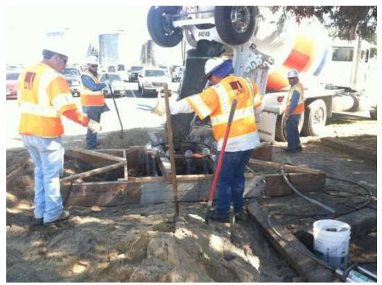
Figure 5 – Crews poor concrete for a TSP foundation adjacent to the Gallo Substation. View east, 02/24/15.
