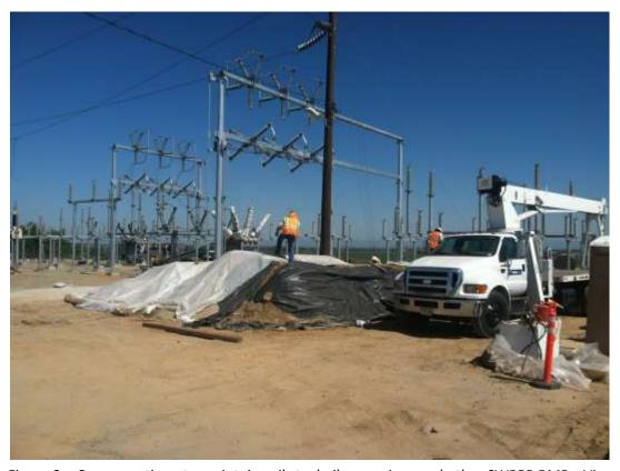
Figure 3 – Crews continue to maintain soil stockpile coverings and other SWPPP BMPs. View northeast, 03/19/15.
