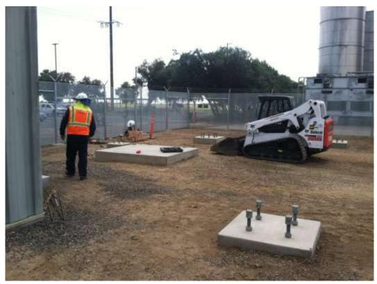
Figure 2 – Crews resumed foundation installation work at the Gallo Substation during the subject period. View southeast, 04/08/15.
