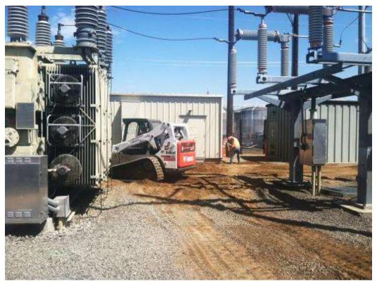
Figure 4 – Crews installed conduit at the Gallo Substation during the subject period. View east, 04/24/15.
