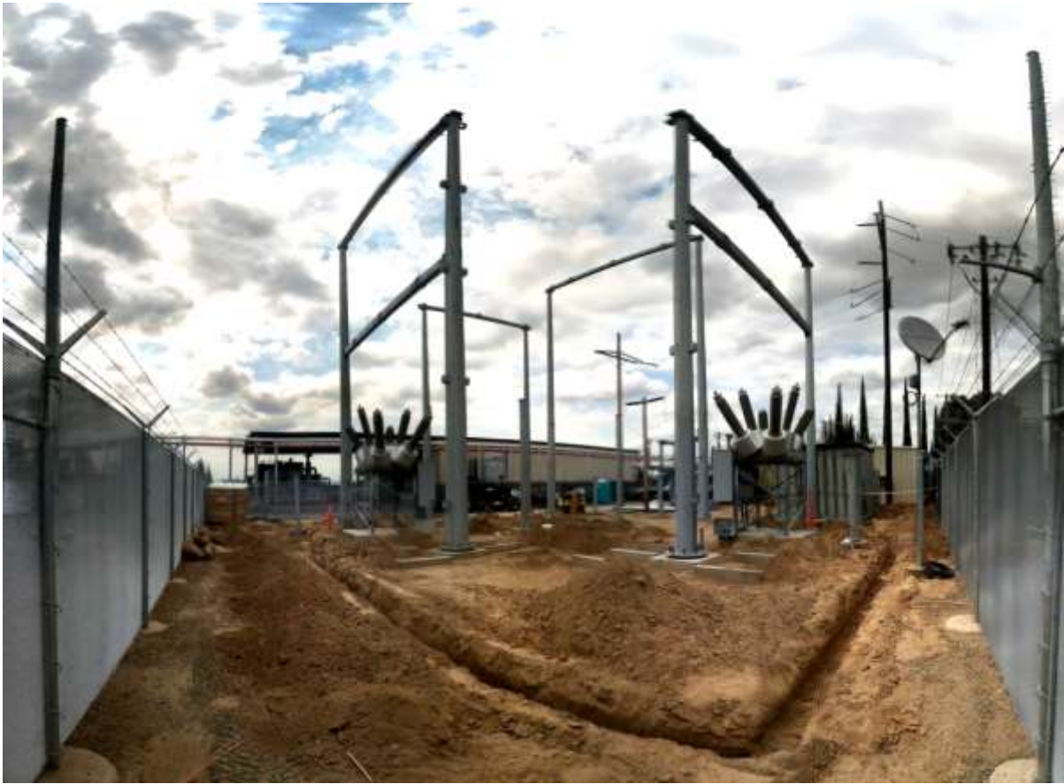
Figure 2 – Work continued at Gallo Substation during the subject period. View northwest, 5/21/15.
