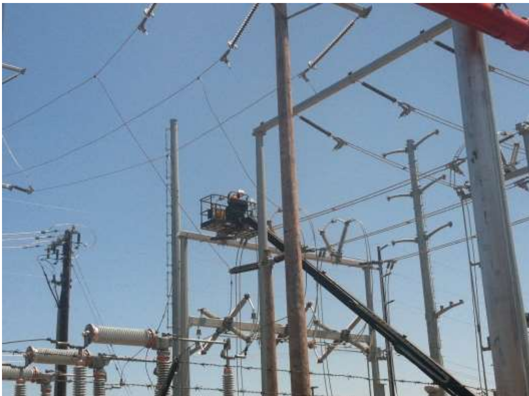
Figure 2 – Crews continued installing structures at the Gallo Substation during the
