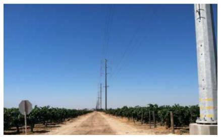
Figure 1 – Removal of the Shoo-Fly (left row of poles and line) was completed during the subject period. View north, 6/26/15 above, 6/30/15 middle, 7/29/15 below.
