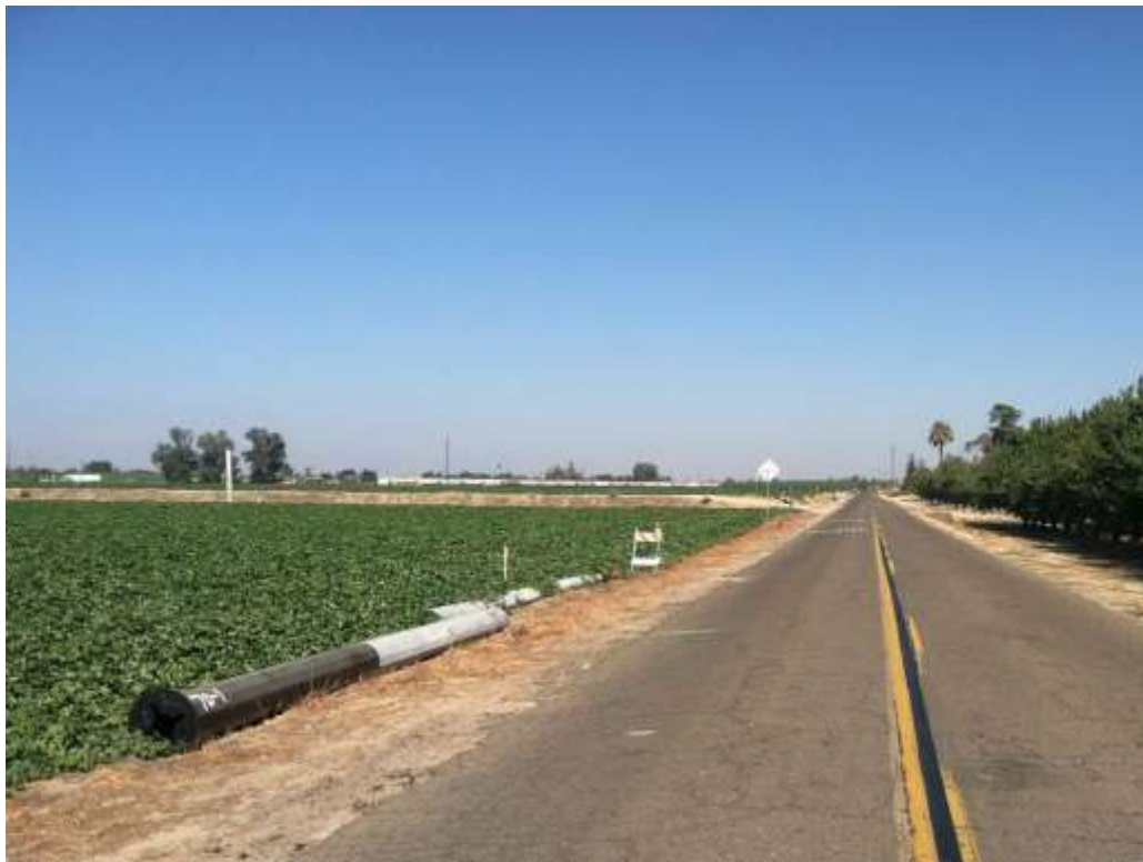
Figure 2 – Poles remain staged along Magnolia Avenue for installation in the coming weeks. View east 8/19/15.
