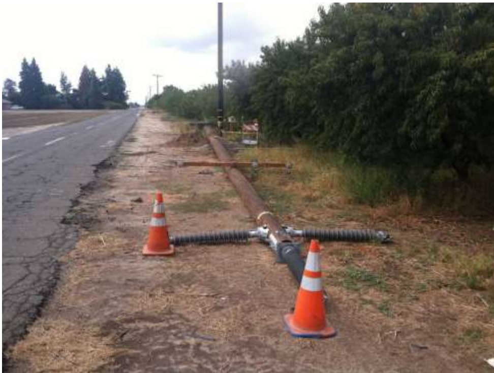
Figure 2 – Poles remain staged along Magnolia during the subject period. View west 10/1/15.
