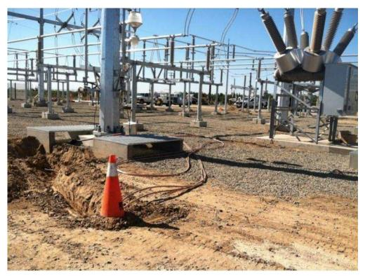
Figure 1 – Grounding wires were installed at the Cressey Substation during the subject period. View southwest (photo provided by PG&E).
