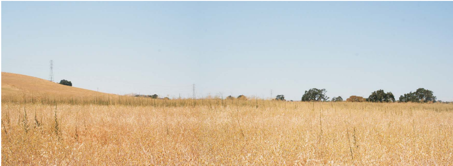
Project Site, Existing Contra Costa–Cayetano 230kV Transmission Line Towers, looking Northwest
