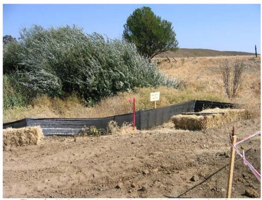
**Figure 3** – Silt fences and other erosion controls in place near Sand Creek. September 12, 2007.
