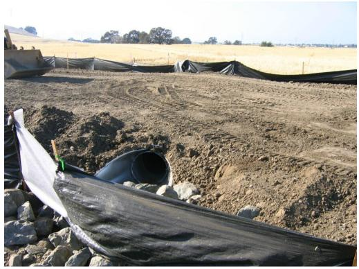
Figure 3 – New culvert installed along access road at wetland area #3, October 31, 2007.
