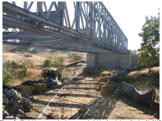
Figure 2 – The bridge structure has been set on the bridge foundations, October 31, 2007.
