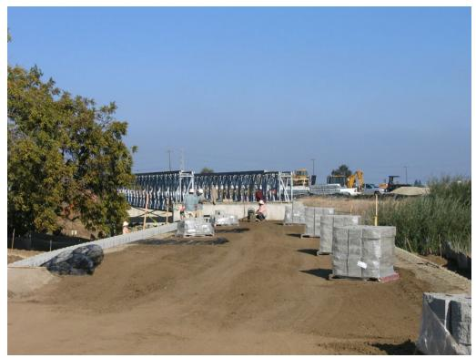
**Figure 1** – Crews working on keystone retaining wall on the south side of Sand Creek, October 31, 2007.
