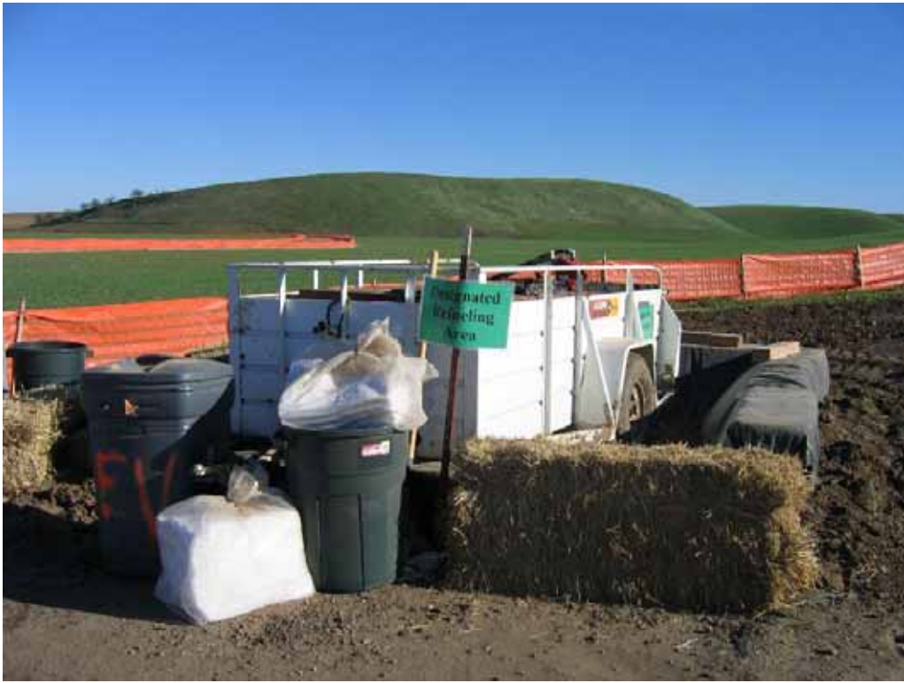
Figure 3 – New designated refueling area at Substation site, February 14, 2008.
