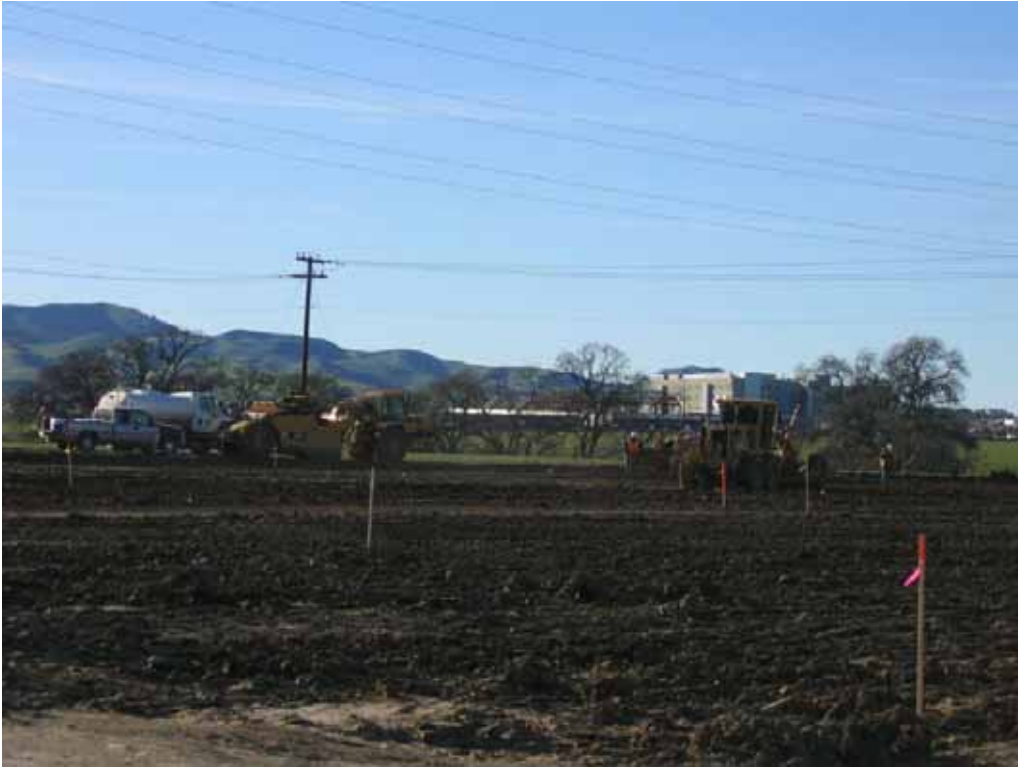
Figure 1 – Crews working at substation grading and compacting fill, February 14, 2008.
