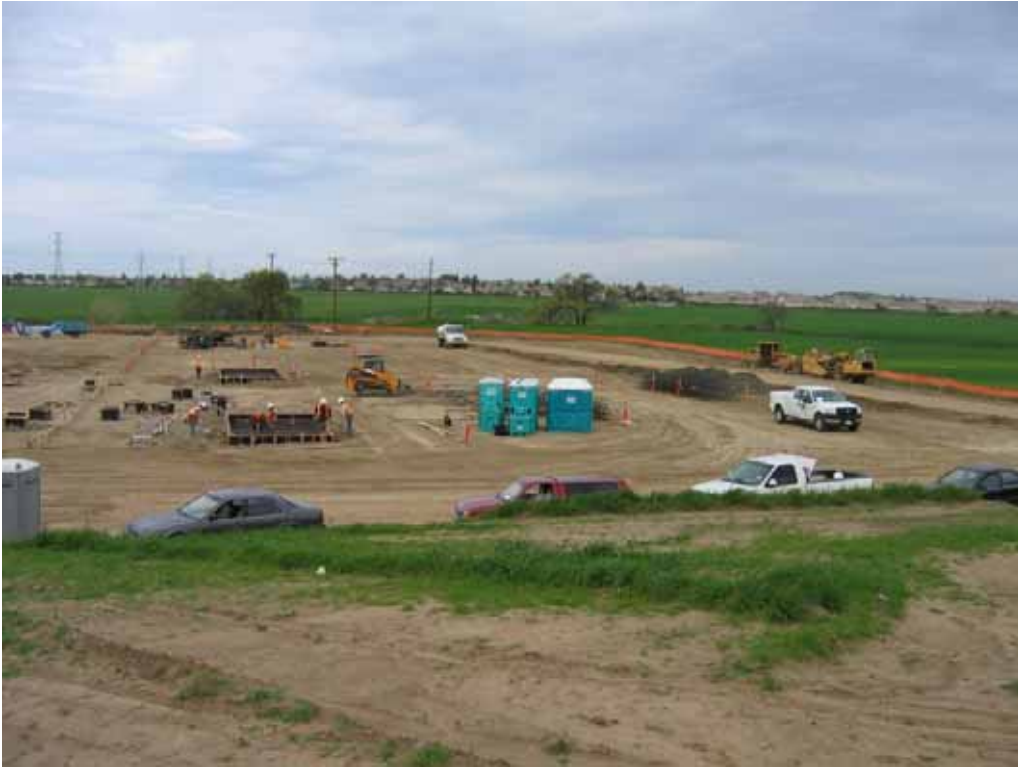
Figure 1 – View of substation site looking north, March 12, 2008.
