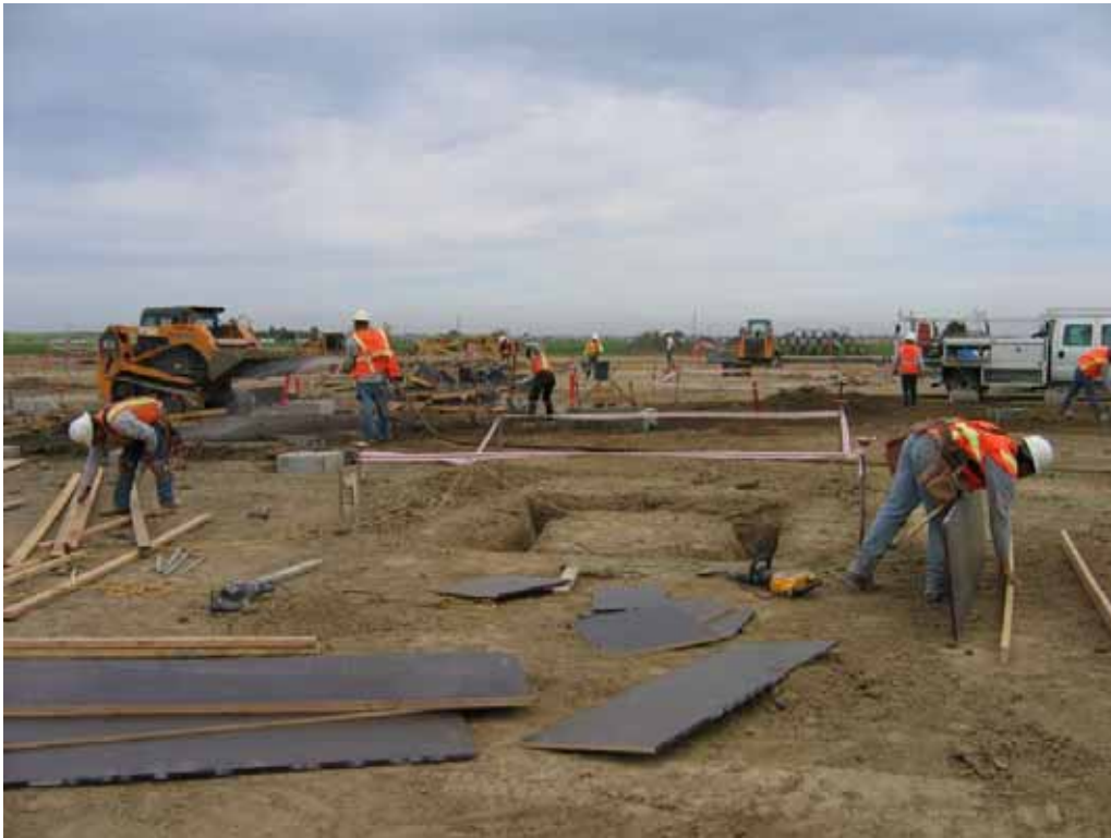
Figure 3 – Crews working on foundation forms at the substation site, March 12, 2008.
