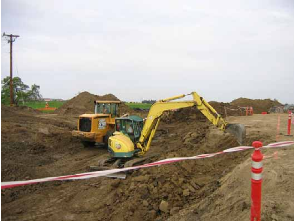
Figure 3 – Crews excavating SPCC pond at the substation site, April 2, 2008.
