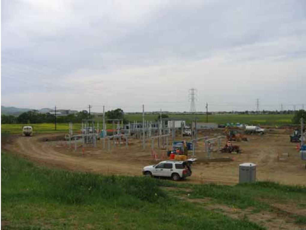
Figure 1 – View of substation site looking northwest, April 2, 2008.
