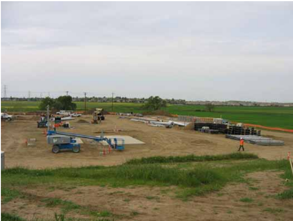
Figure 2 – View of substation site looking northeast, April 2, 2008.
