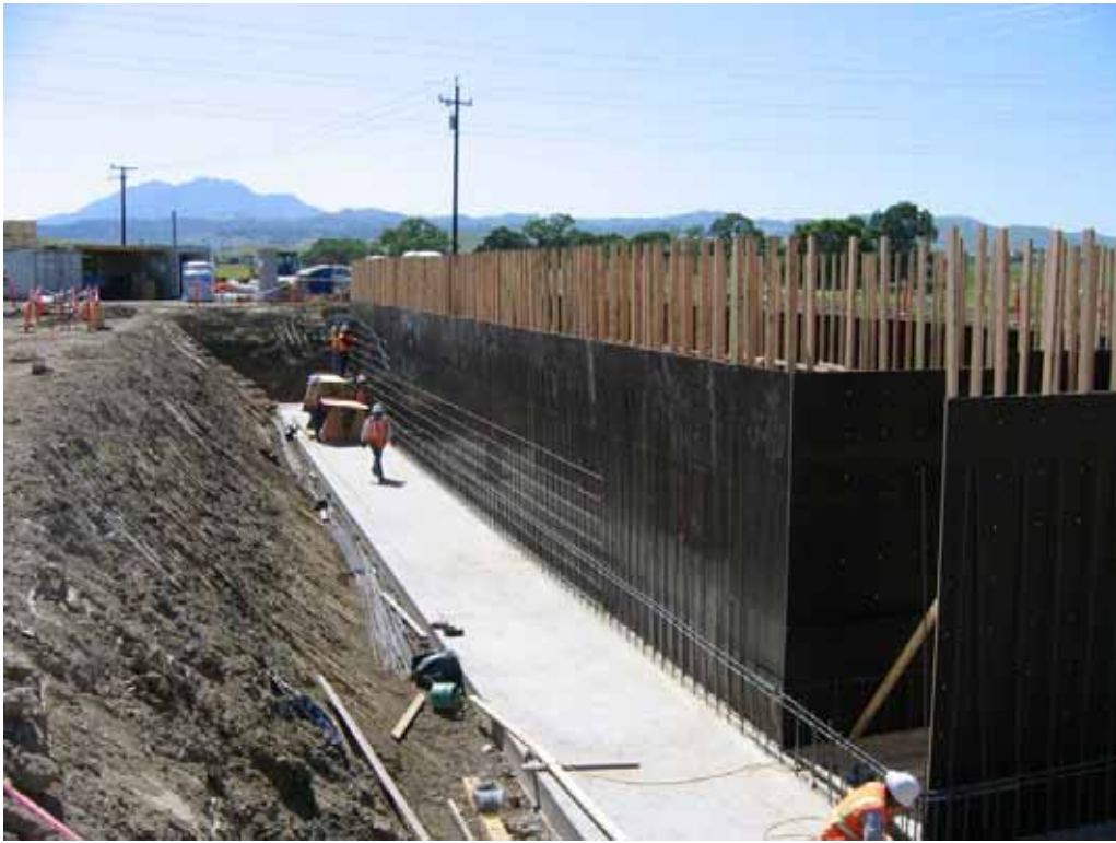
Figure 3 – Constructing forms for the SPCC pond, April 17, 2008.
