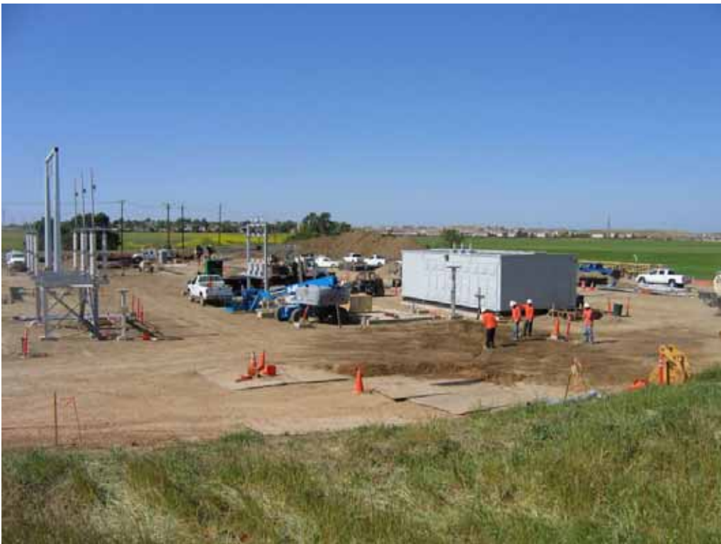
Figure 2 – View of substation site looking northeast, April 17, 2008.
