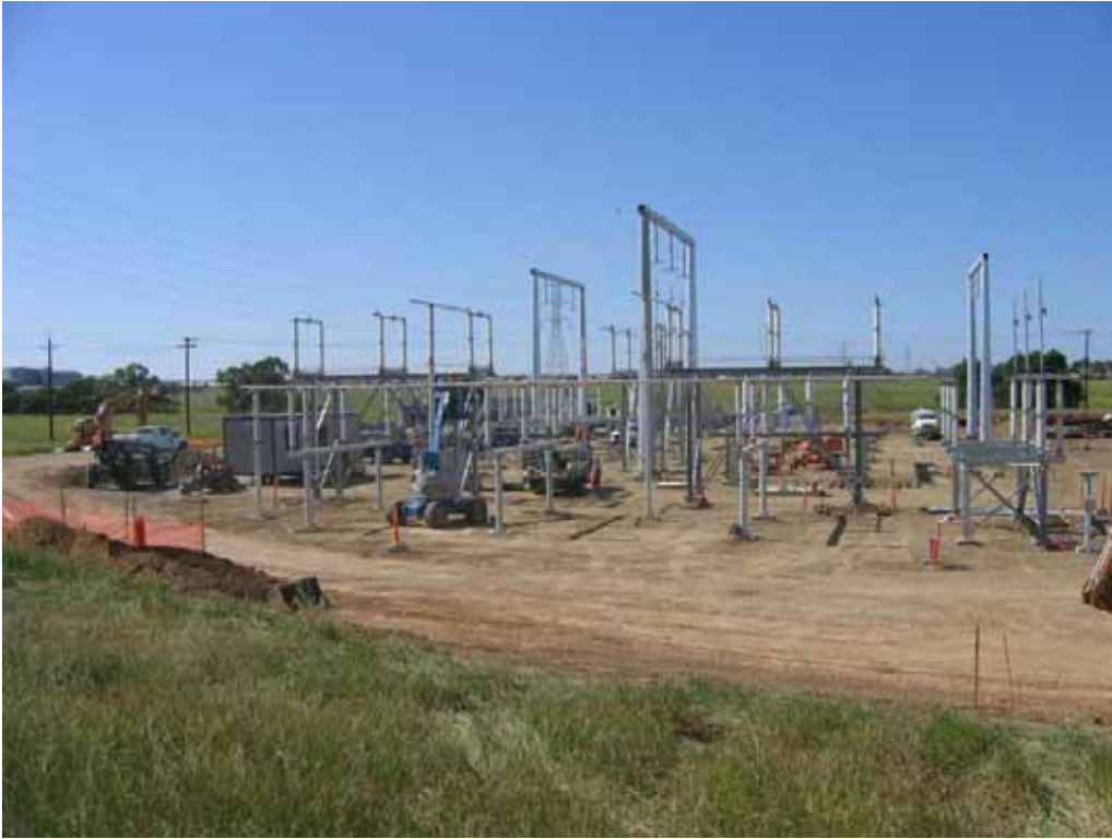
Figure 1 – View of substation site looking northwest, April 17, 2008.
