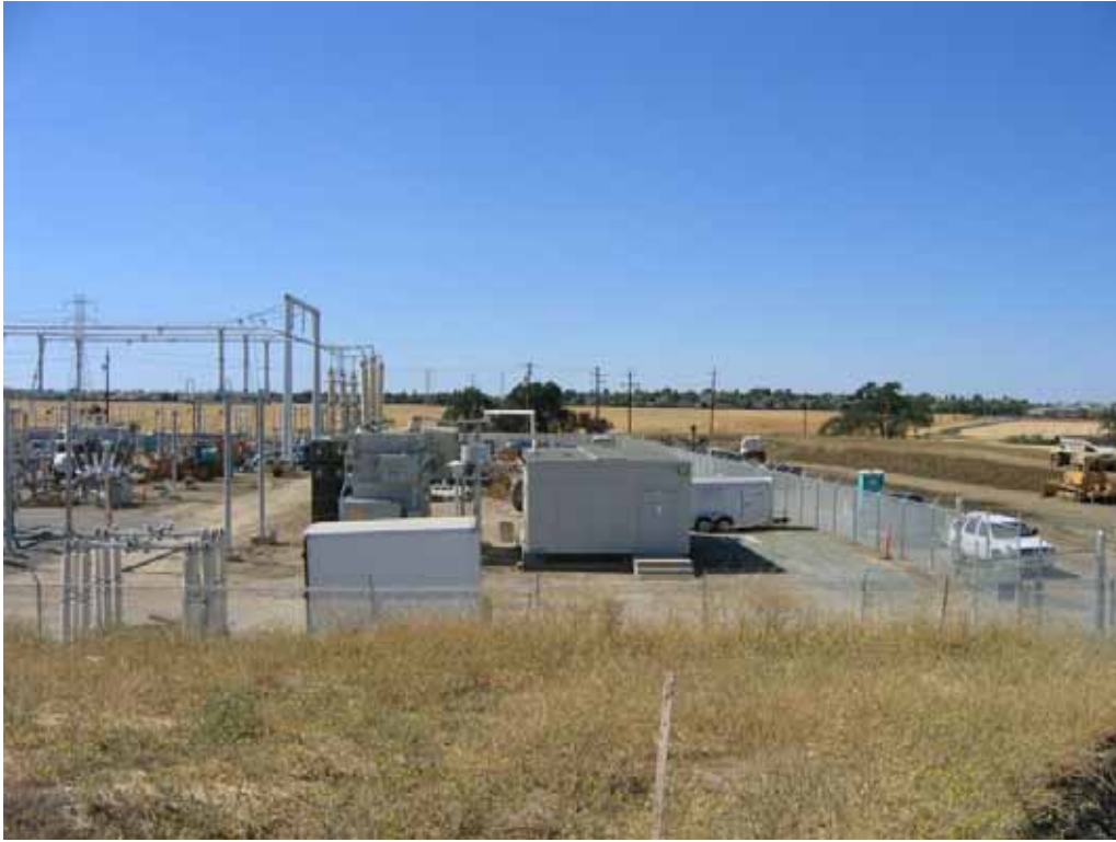
Figure 3 – Substation site looking northeast, 2008.
