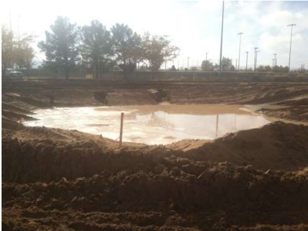
Figure 6 –Evidence of flow entering into the work area from offsite during the week’s rain. No onsite sediment was transported offsite. View south, December 4, 2014.
