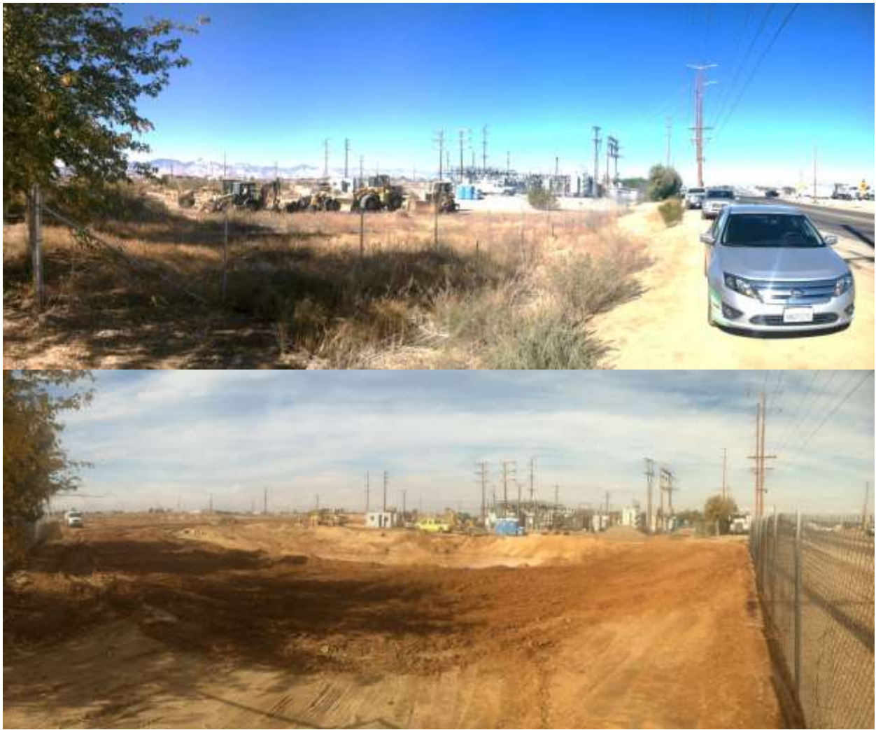
Figure 3 – Panoramic view of grading from southeast corner of site. Fence-line has moved outward along eastern boundary to accommodate necessary grading. View northeast, December 4, 2014.
