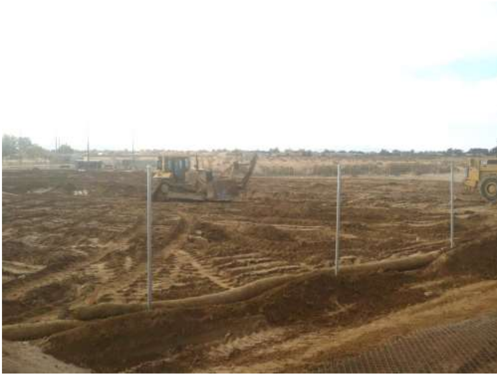
Figure 1 – Grading continued. View southwest, December 4, 2014.
