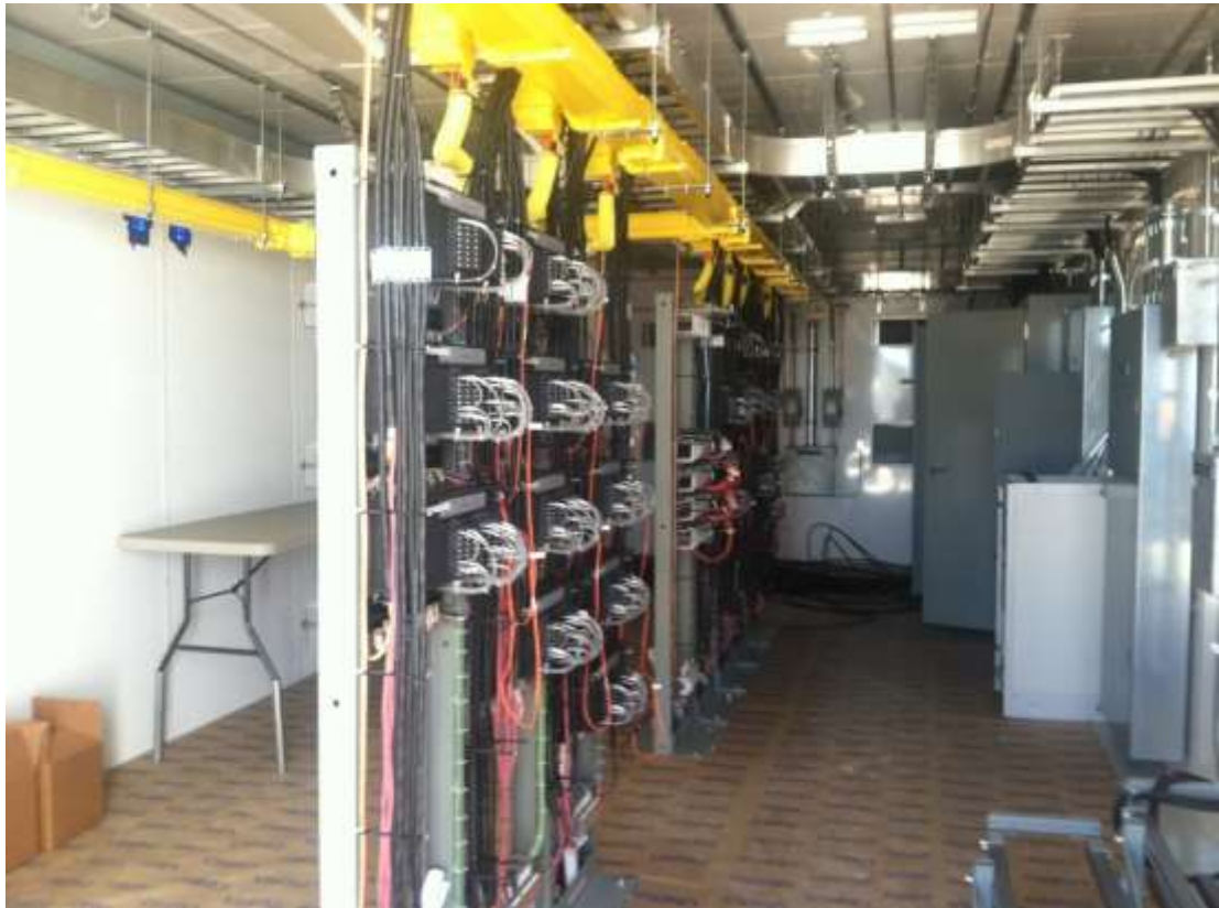
Figure 4 – Installation of the MEER building continued. View west, 02/12/15.
