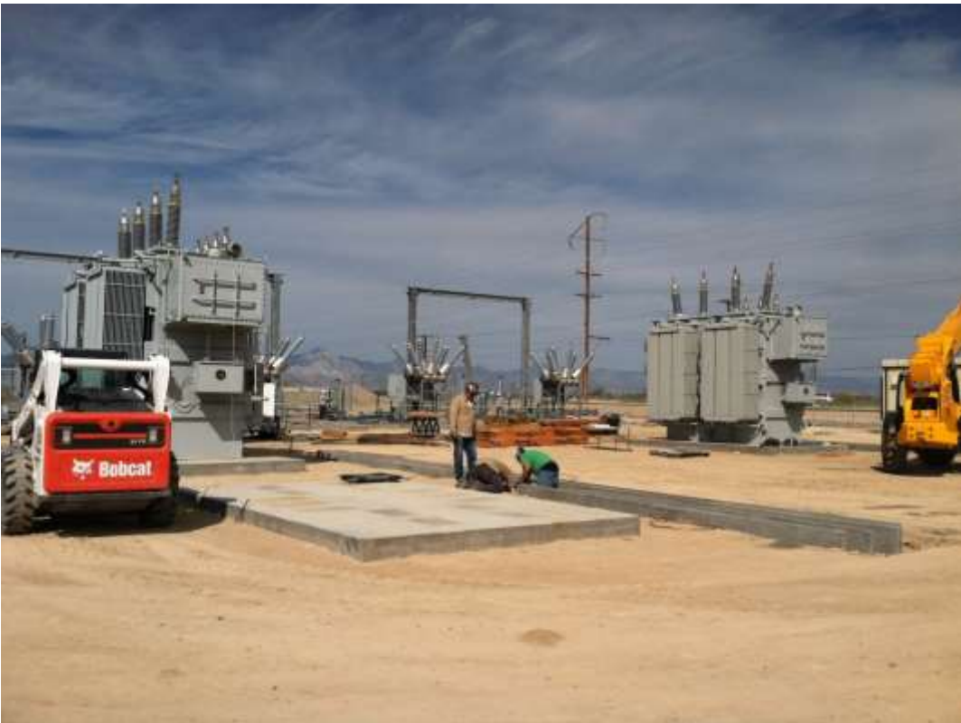
Figure 3 – Trenching work continued during the subject period. View northwest, 03/17/15.
