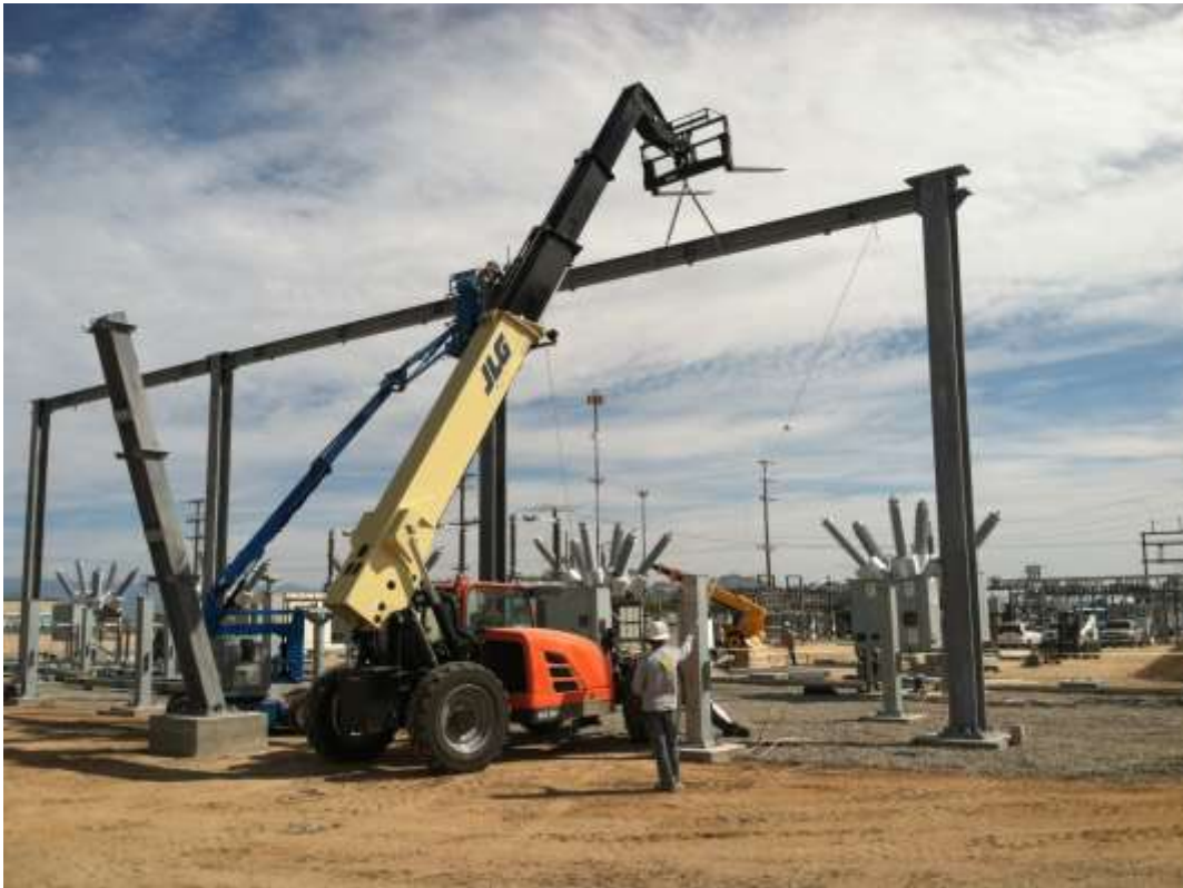
Figure 2 – Structure installation occurred during the subject period. View northeast, 03/17/15.
