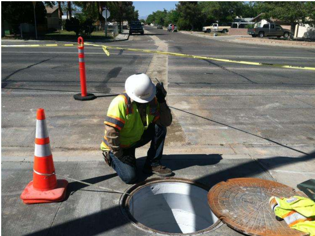
Figure 3 – Fiber optic work was completed at the SCE Ridgecrest Service Center during the subject period. View north, 04/13/15.
