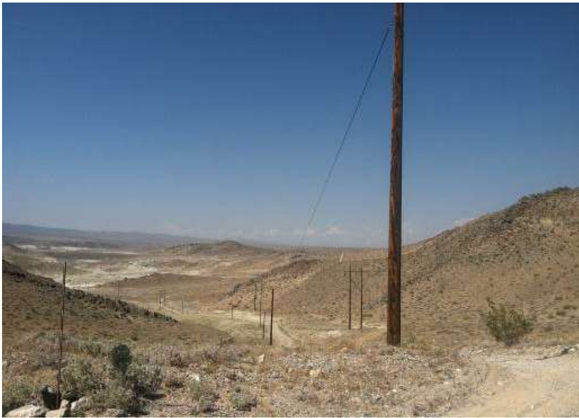
Figure 5 – Linear work continued during the subject period. View southwest, 4/13/15.
