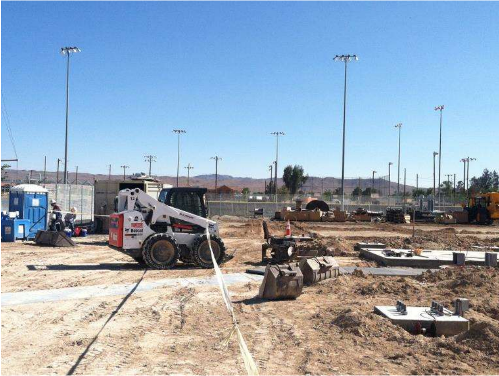
Figure 1 – The Downs Substation pad remains 60% complete. View south 04/13/15.
