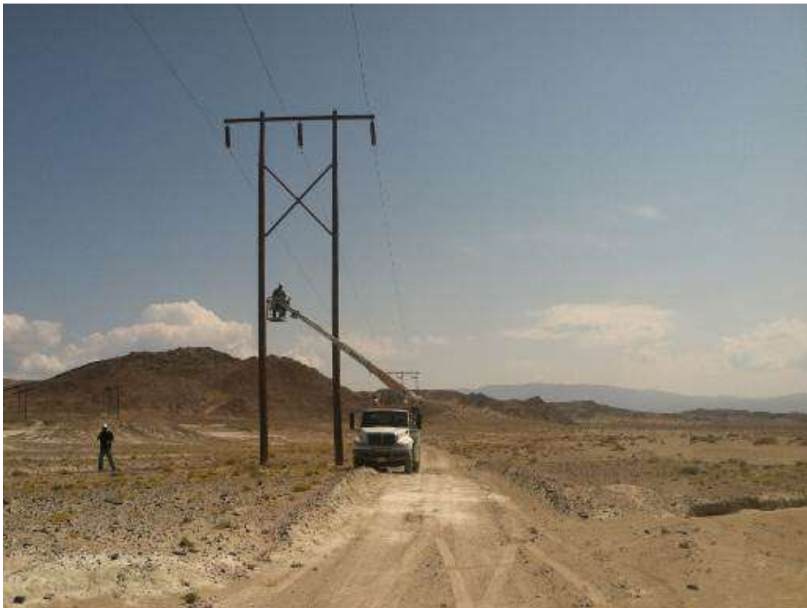
Figure 6 – Linear work continued during the subject period. View northeast, 4/13/15.
