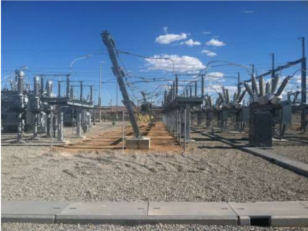
Figure 1 – Installation of interior fencing occurred during the subject period. View south, 6/11/15.
