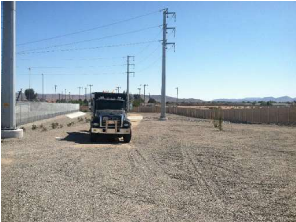
Figure 2 – Some additional structure demolition work is anticipated. View south 04/4/16.
