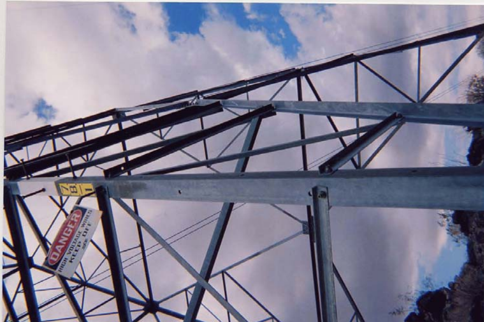
8-3-2006 -DPV1 Tower No. 78-1 off Pipeline Rd. in the Kofa Nat'l Wildlife Refuge, Az. near the western end of the manmade scarring.
