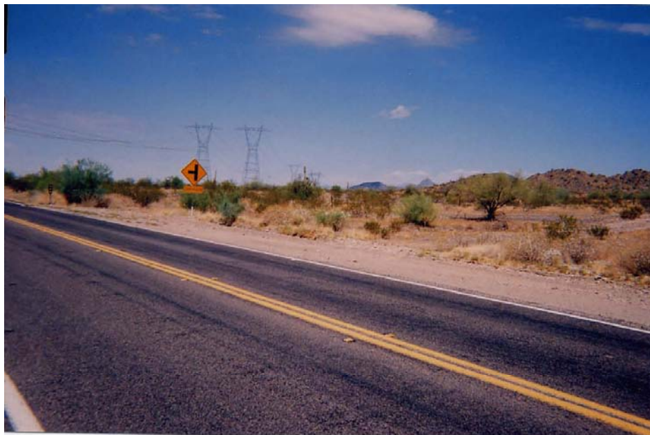
8-3-2006 - Salome Rd. view looking NW (before Courthouse Rd. Intrsctn at the DPV1 & Harq. Hassayampa adjacent 500kV Lines in Harquahala Valley, Az.
