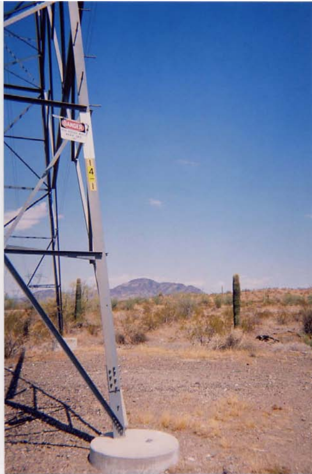
8-3-2006-DPV1 Tower No. 14-1, the first tower on the right side of Salome Hwy., N. of Intersection w/Courthouse Rd., Harquahala Vly., Az; tower very close/adjacent #5-2
