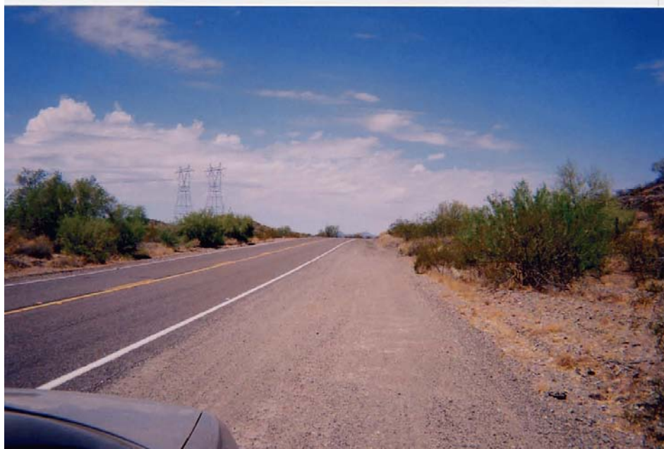
8-3-2006 - driving westerly on Salome Hwy before reaching Harquahala Vly, DPV1 & Harq.-Hassayampa 500kV Towers southeast of the Intersection with Courthouse Rd.
