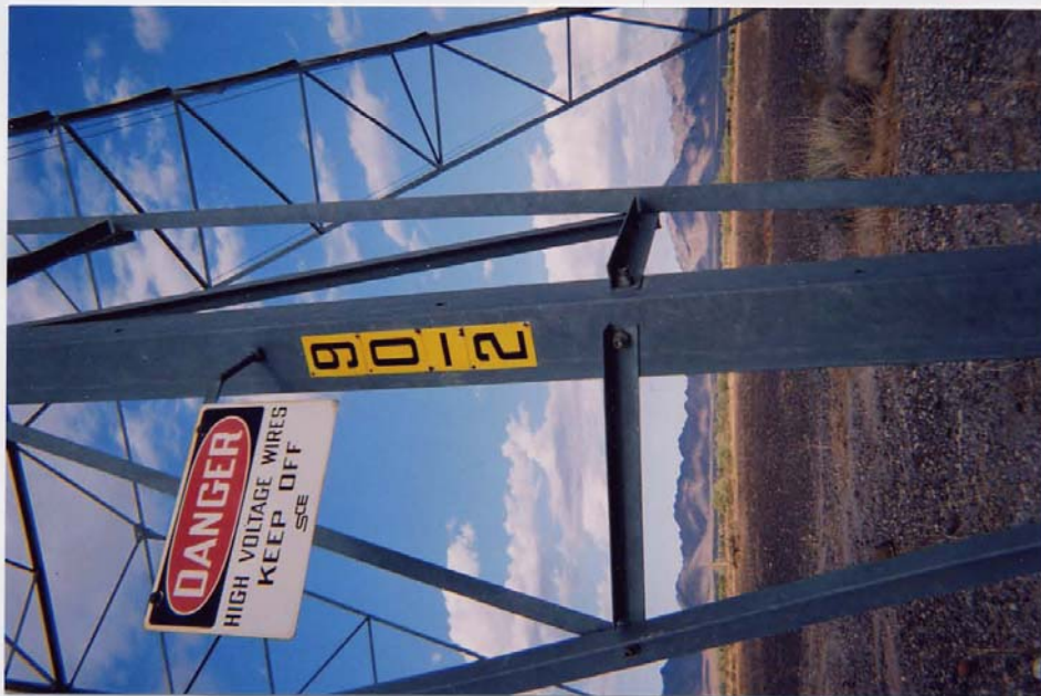
8-3-2006 - the DVP1 Tower, the first, west of US95 in Az. is Tower No. 90-2
