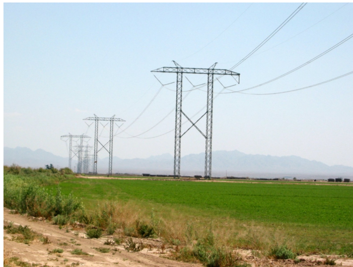
Photo 3 - 500 kV H-Frame towers in agricultural land
