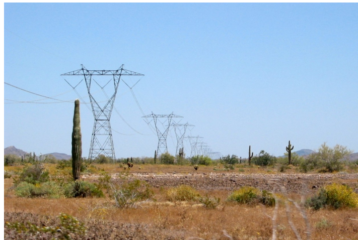
Photo 2 - 500 kV Lattice steel towers east of Highway 95
