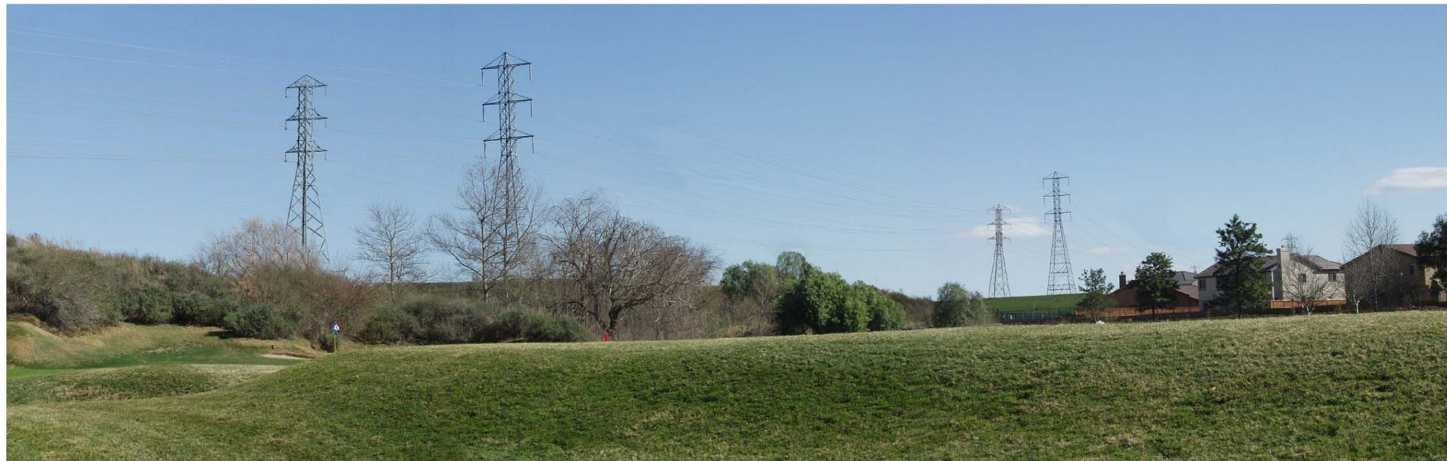
Simulation - Transmission line corridor with two 230kV single-circuit towers (lattice and H-frame) removed and proposed 230kV double-circuit lattice steel structure transmission line.
