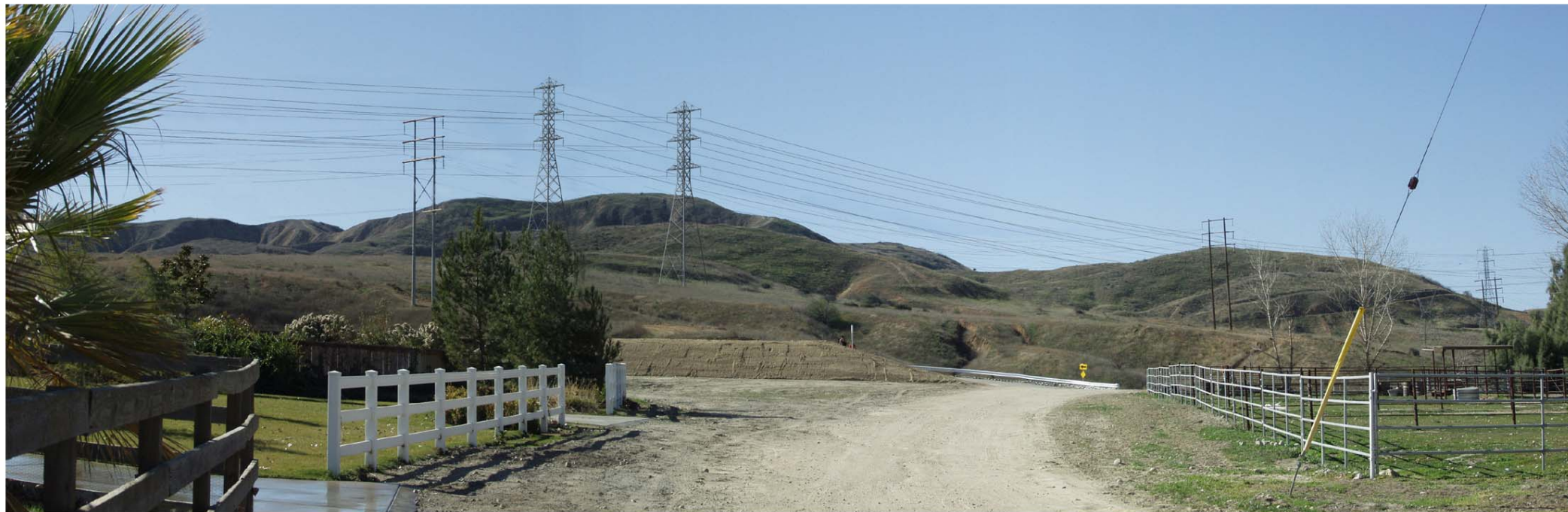
Simulation - Transmission line corridor with two 230kV single-circuit lattice towers removed and proposed 230kV double-circuit lattice steel structure transmission line.
