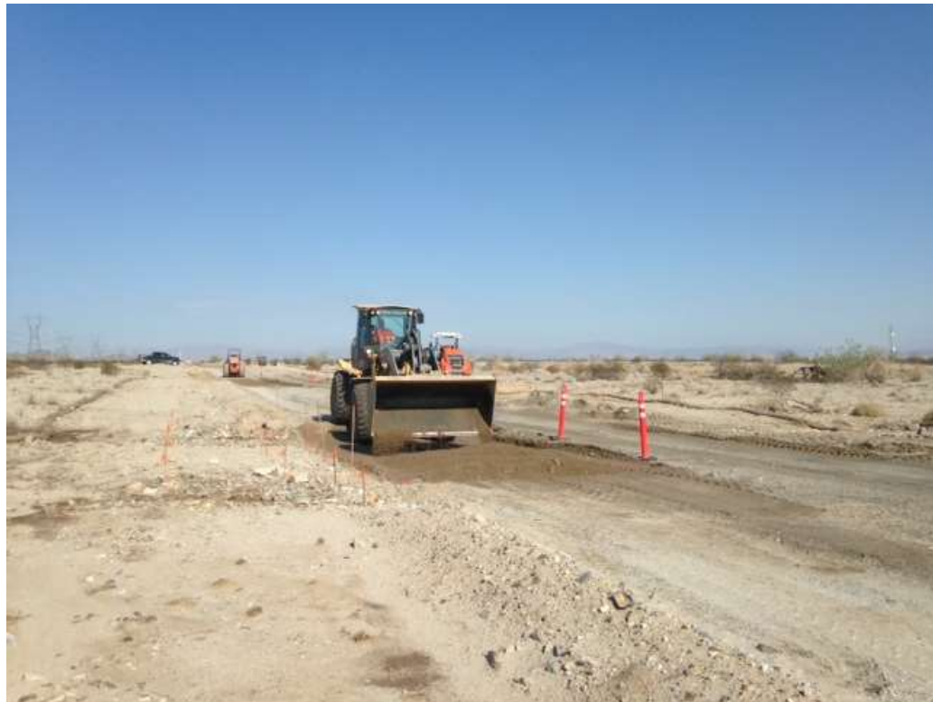
Figure 2. Grading activities along the access road.
