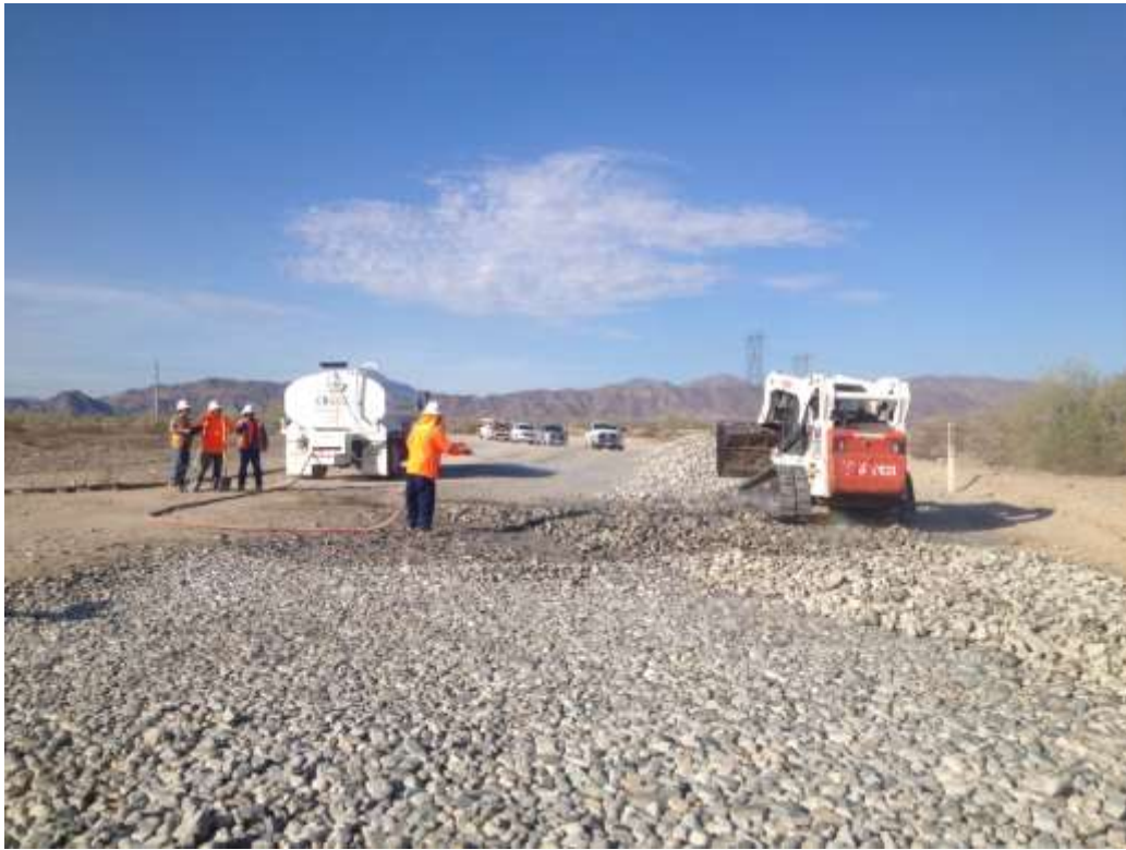
Figure 1. Construction entrance stabilization (Photo courtesy of FRED).
