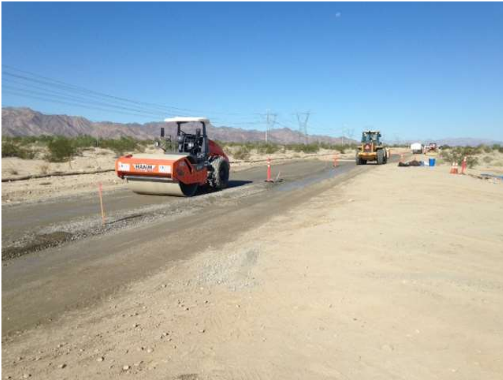
Figure 1. Access road compaction between Arizona Crossings.
