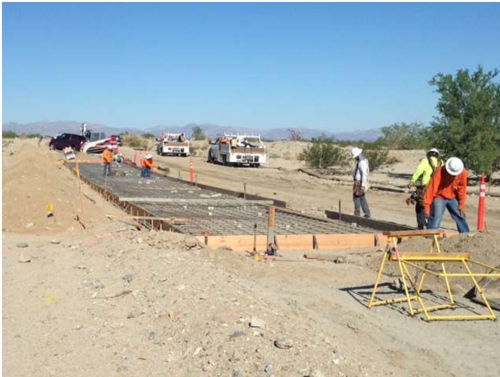
Figure 2. Setting rebar and forms for an Arizona Crossing.
