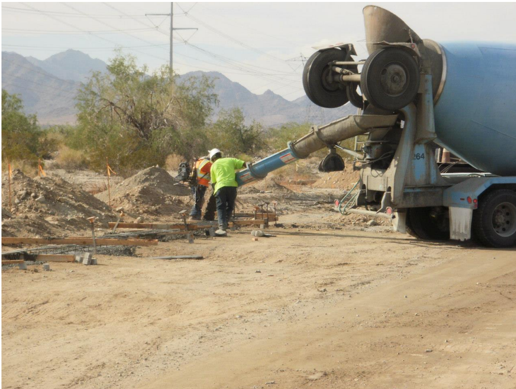
Figure 2. Pouring concrete footers for Arizona crossing
