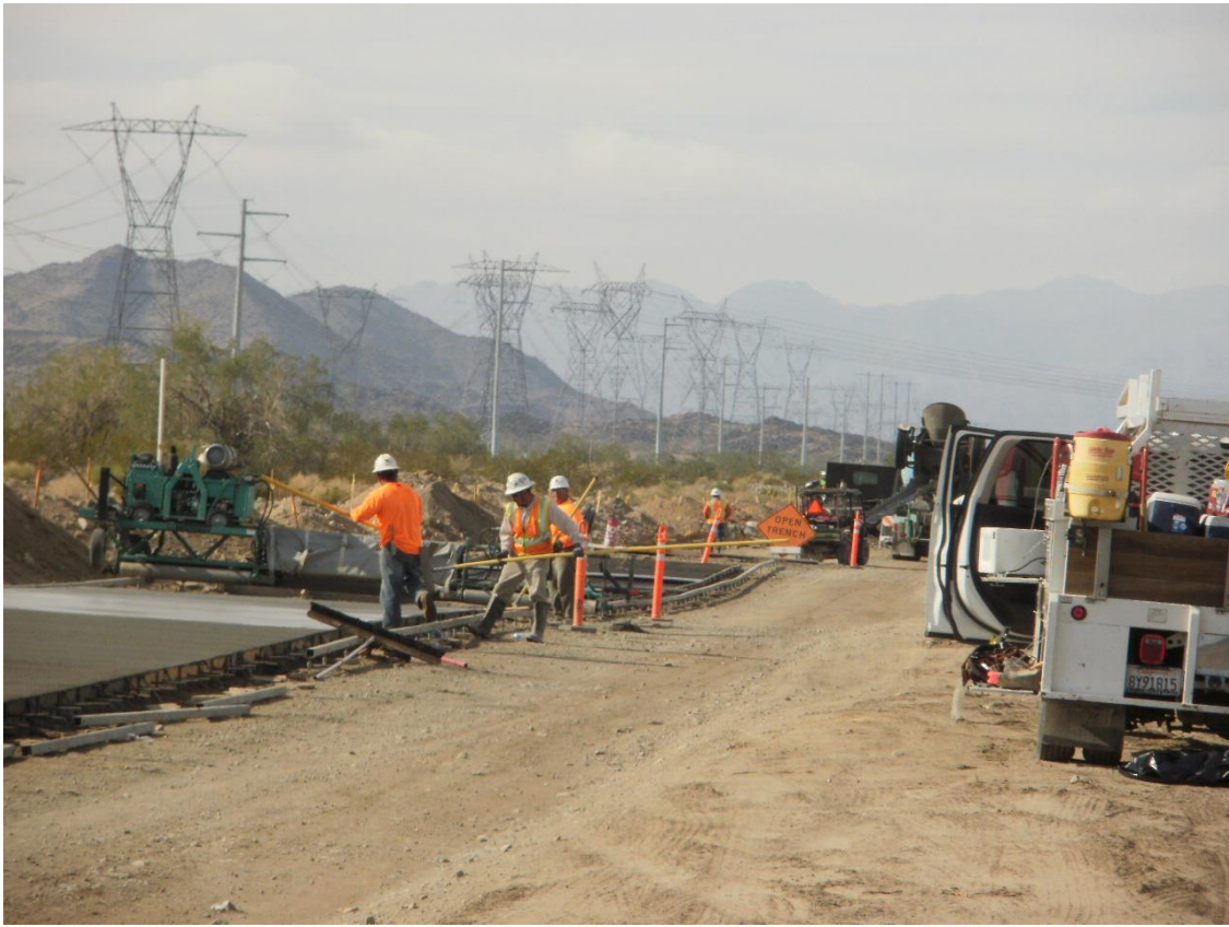
Figure 3. Smoothing concrete for Arizona crossing
