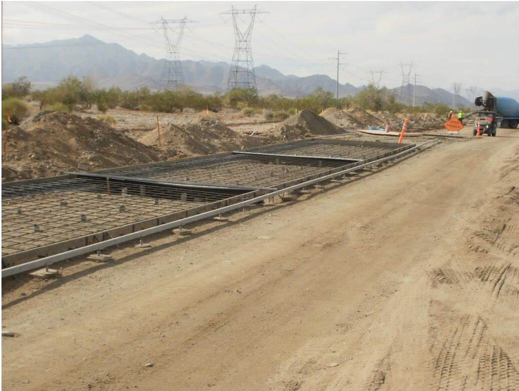
Figure 1. Rebar and forms for Arizona crossing
