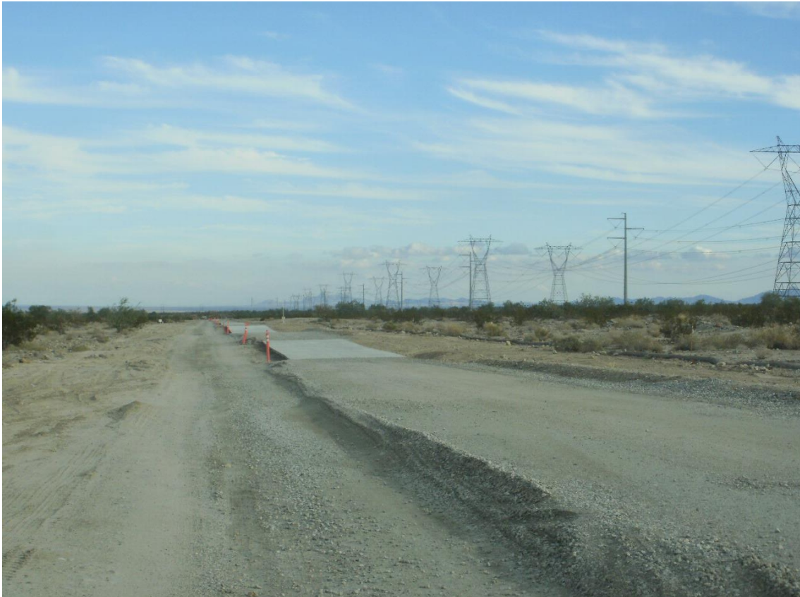
Figure 4. Completed roadway (south side) with Arizona crossings
