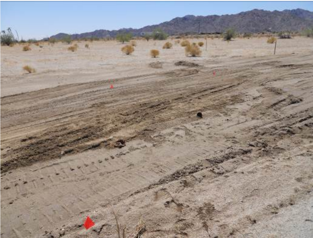
Figure 8: Potential cultural resource (can scatter) was identified during grading. Note pin flagging to delineate avoidance area until consultation with project archaeologist. Archaeologist later determined no cultural/historical significance.
