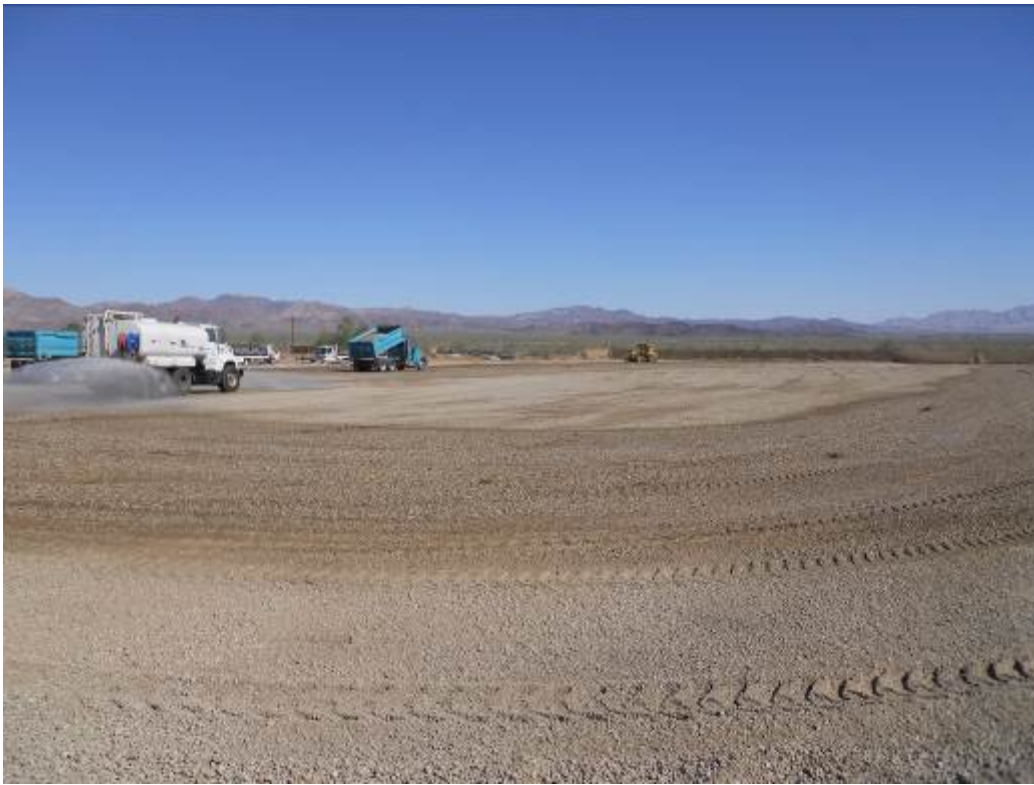
Figure 7: Gravel placement and dust abatement activities occurring at DC1.
