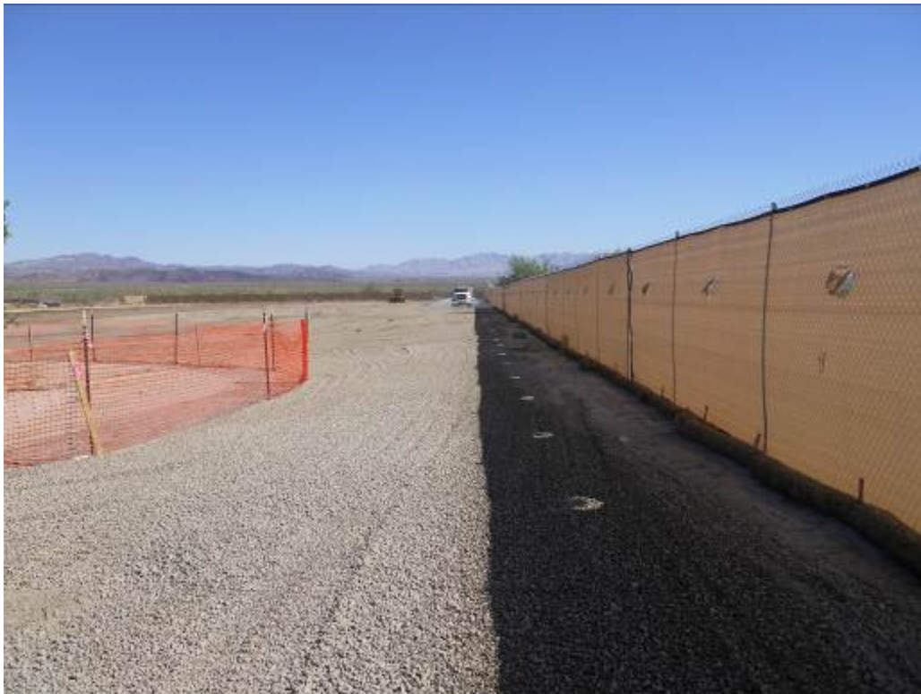
Figure 2: Privacy screening installed along east fence line at DC1.
