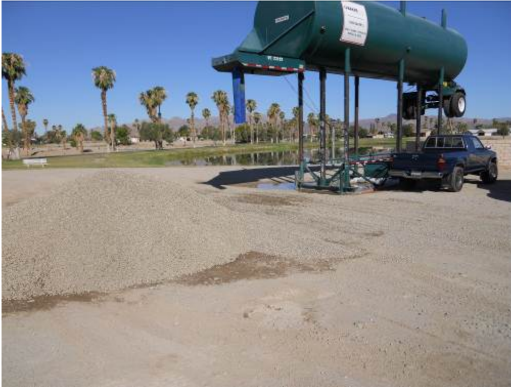
Figure 1: Baker tank installed at water resource location north of DC1 and DC2.
