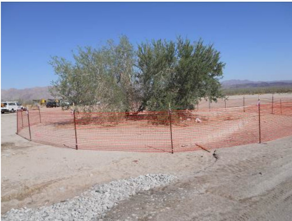
Figure 6: Orange construction fencing identifying nest buffer limits in southeast corner of DC1.
