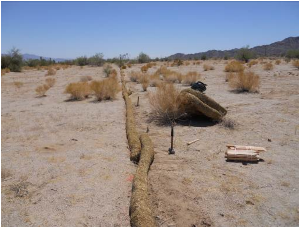
Figure 4: Installation of straw wattles being conducted at DC2.
