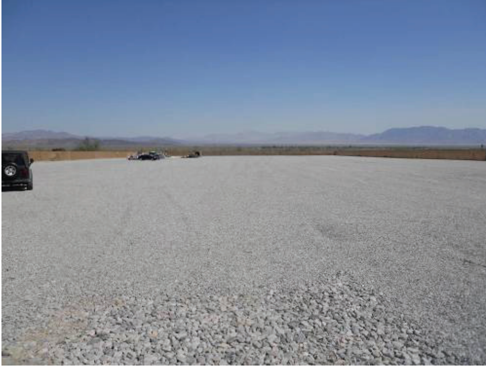
Figure 1: Construction activities completed at DC1 Yard. View north from yard entrance.
