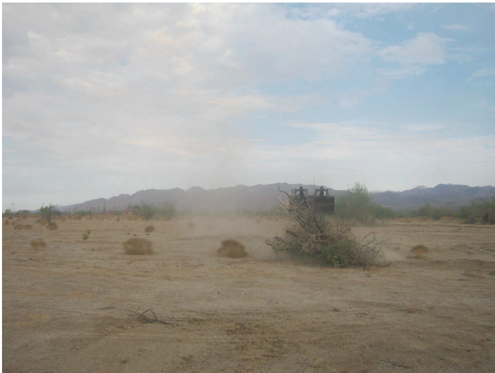
Figure 4: Excessive dust during tree removal activities at DC2.
