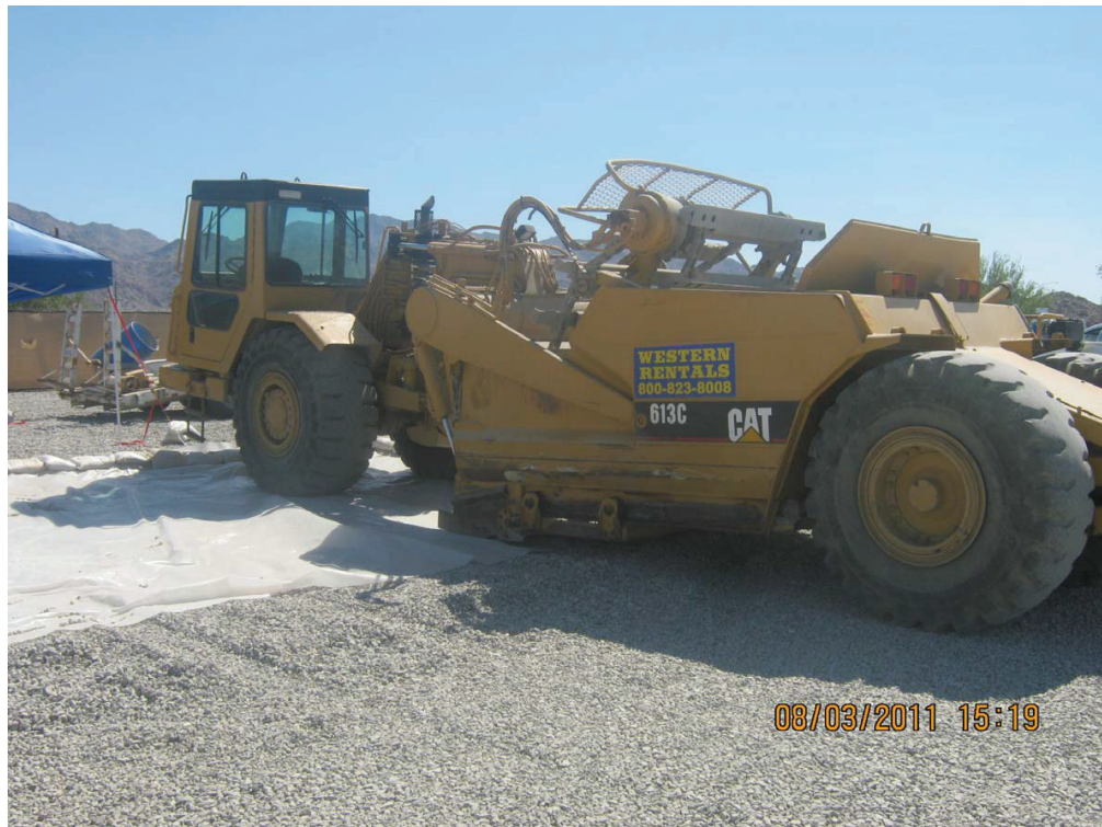
Figure 4: Equipment improperly parked at DC2 with only partial coverage of plastic sheeting underneath.
