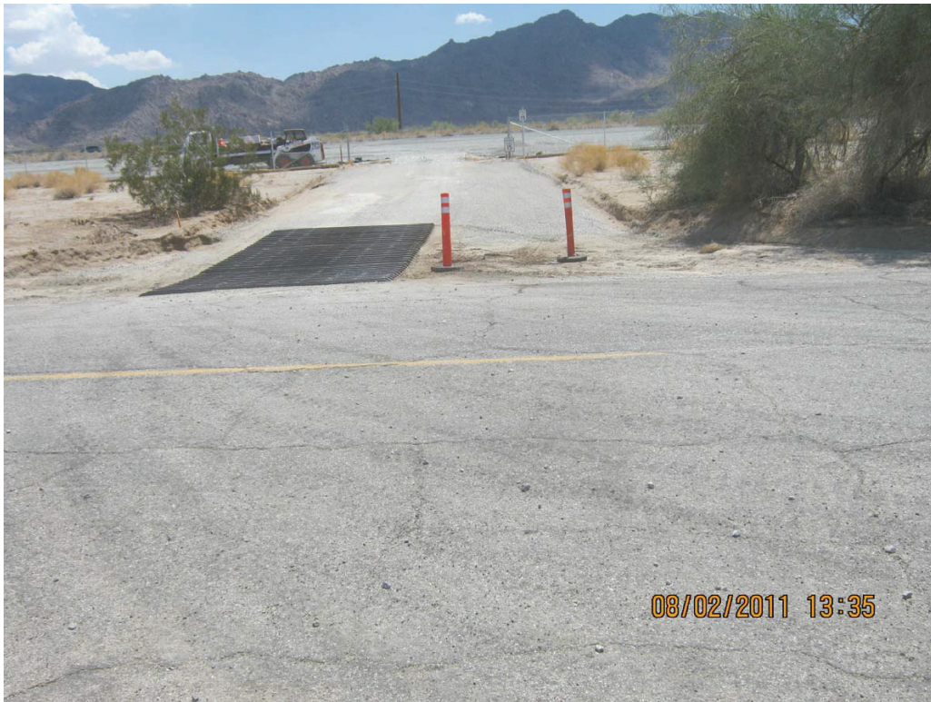
Figure 3: Trackout observed at DC2 (note gravel in foreground).
