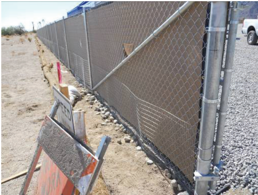
Figure 2: Exclusionary and project boundary fencing has been installed at DC2.
