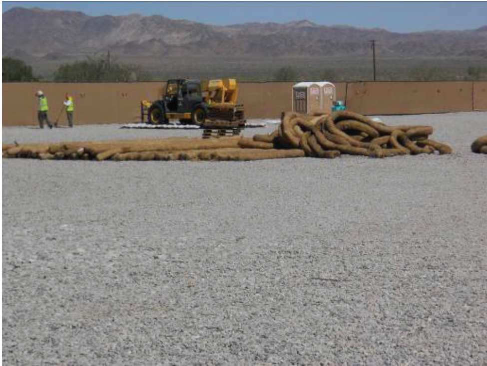
Figure 1: Activities at DC1 included storage of equipment, removal of straw wattles, and localized leveling of gravel.
