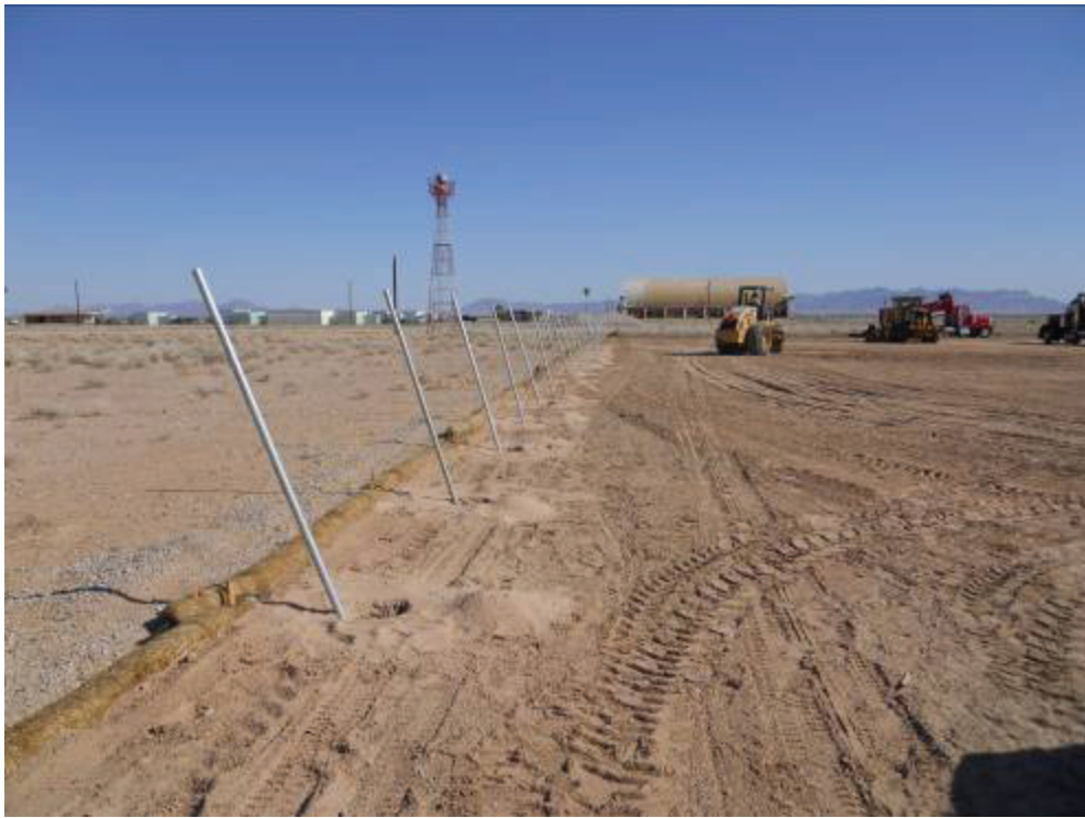
Figure 3: Fence post installation at the Blythe Construction Yard.
