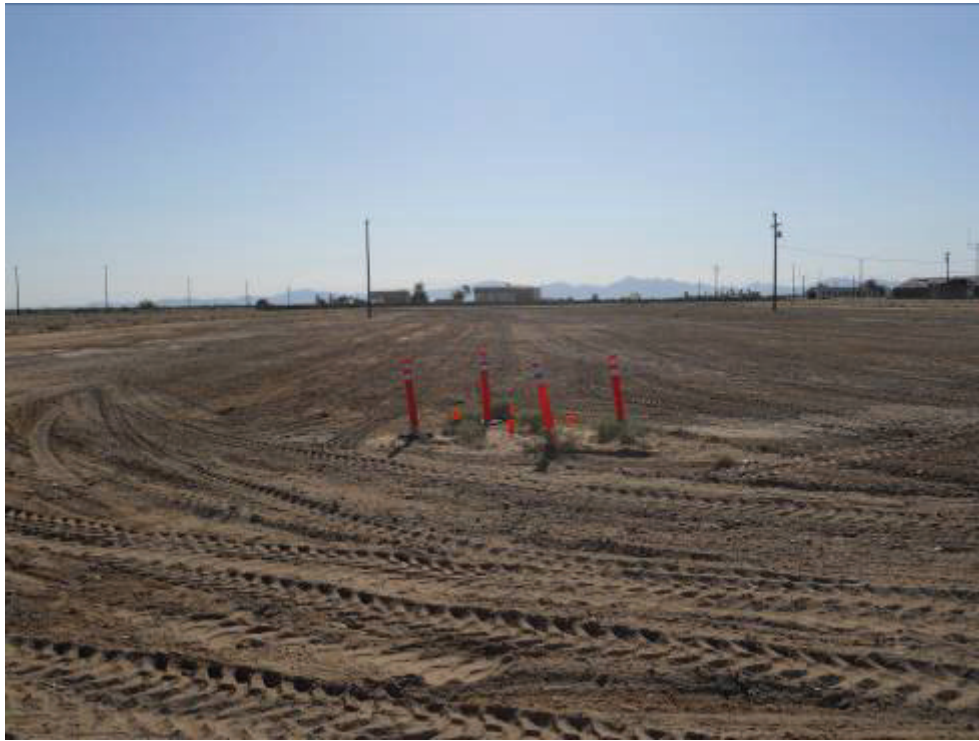
Figure 7: Orange pylons placed at known Harwood's milk-vetch locations at Blythe Construction Yard. Note pin flags that had been installed the previous week.
