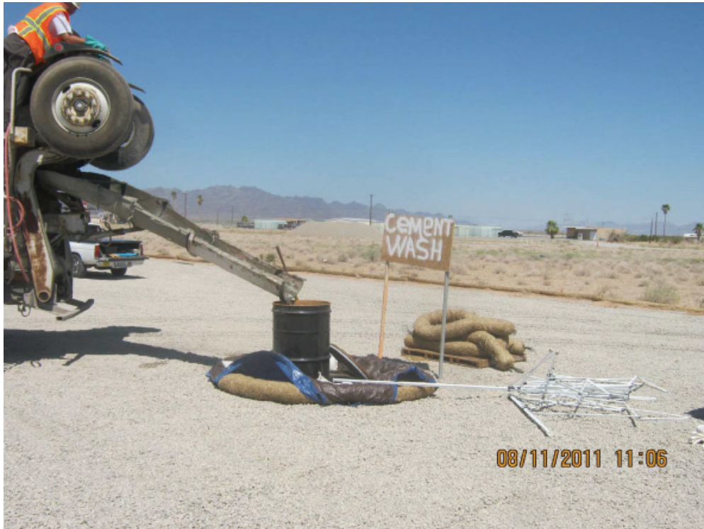
Figure 8: Concrete wash out station being utilized at Blythe Construction Yard.
