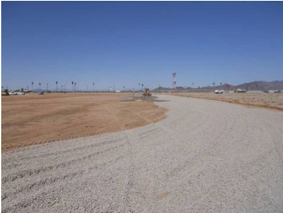
Figure 2: Gravel placement activities at the Blythe Construction Yard.
