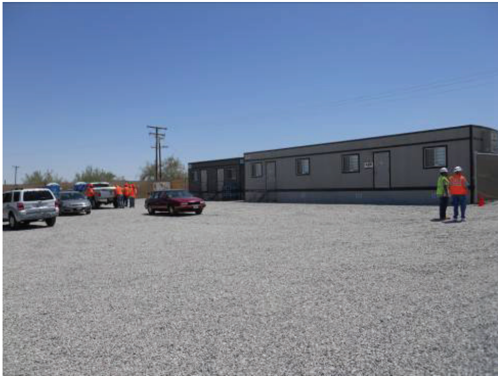
Figure 3: Office trailers have been delivered and completed at DC1 Construction Yard.
