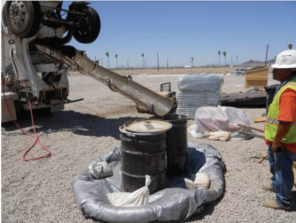
Figure 6: Concrete washout station being utilized at the Blythe Construction Yard.
