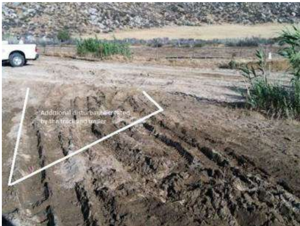
Figure 6. Impacts outside of the approved access road and disturbance area near GS54 (Photo courtesy of FRED)
