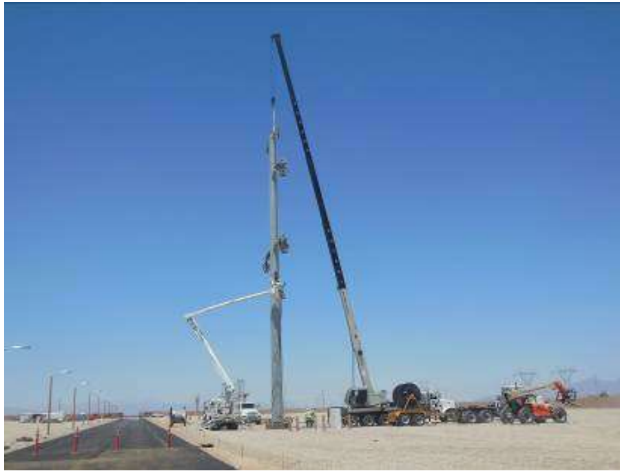
Figure 7. Erection of TSP at CRS.
