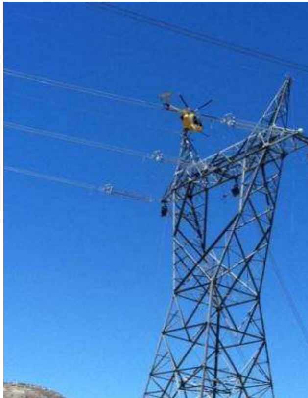
Figure 2. Helicopter wire stringing activities at Tower 1075
