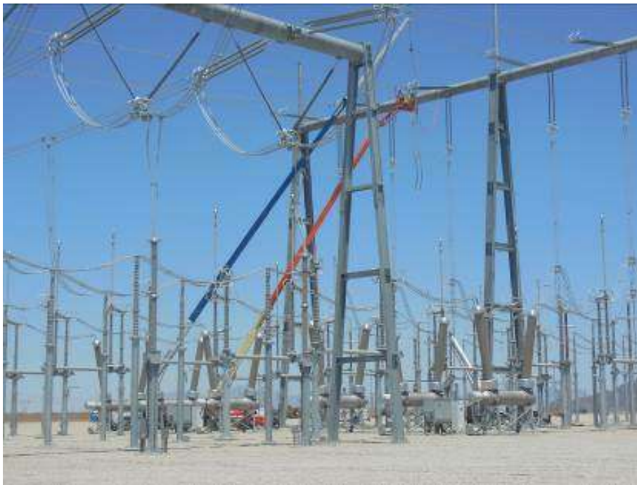
Figure 8. Cable pulling between switchracks at CRS.
