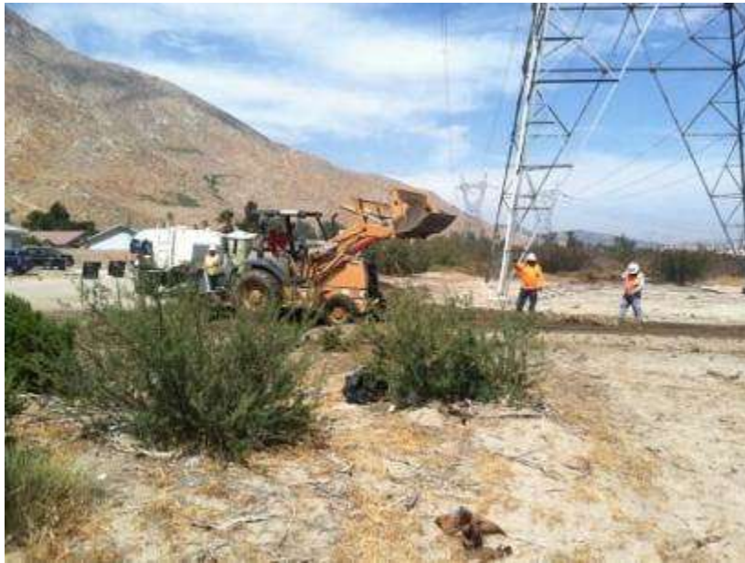
Figure 3. Site stabilization activities at Tower 1053
