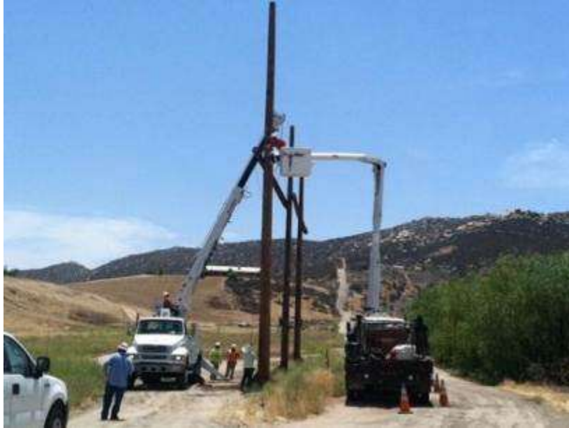
Figure 1. Guard Pole installation at Guard Structure GS60 near Tower 1091
