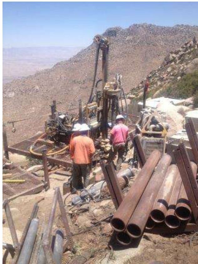
Figure 4. Permanent platform foundation drilling at Tower 1048
