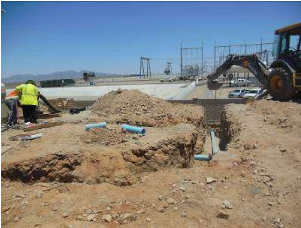
Figure 9. Trenching for permanent water source at Red Bluff.
